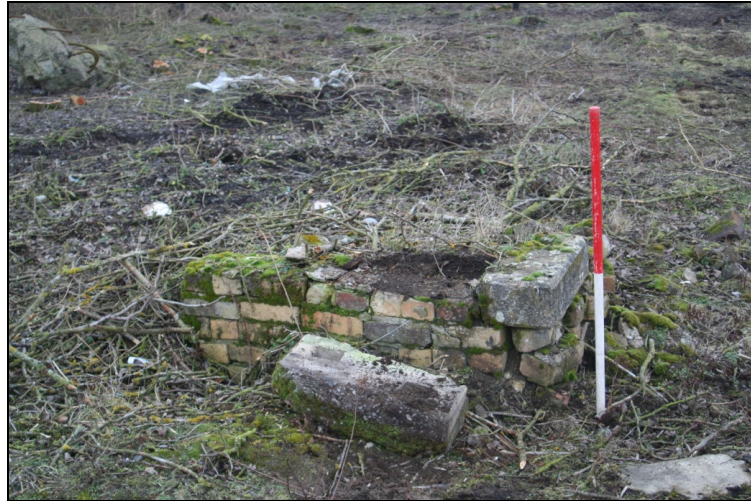
Plate 7. Structure 06 looking east.
