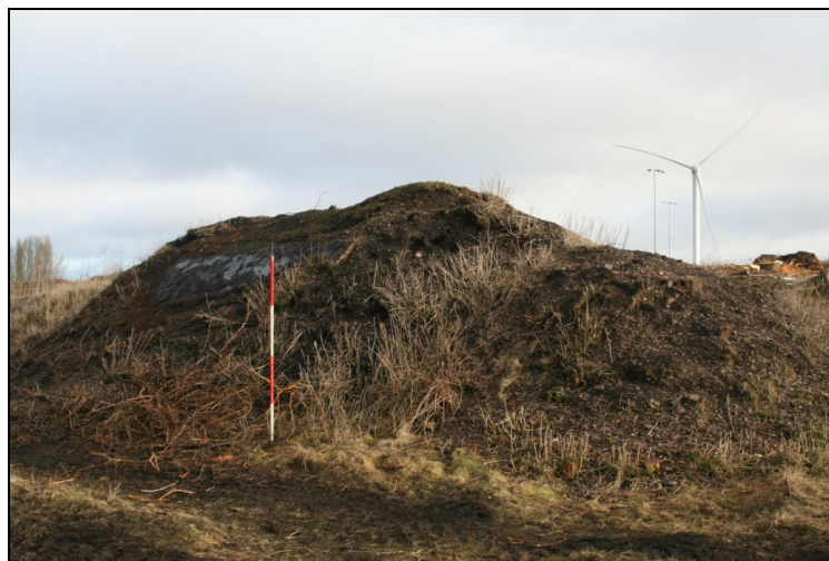
Plate 23. Air Raid Shelter #4 (Structure 24) showing part of the roof, looking northwest
