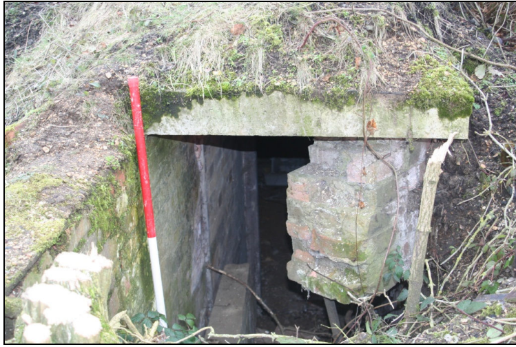
Plate 27. Entrance to Air Raid Shelter #6 (Structure 26) looking west
