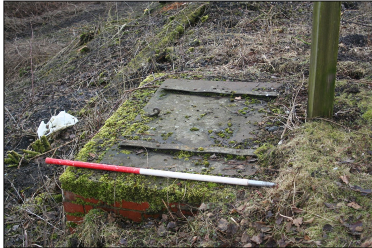
Plate 25. Escape hatch for Air Raid Shelter #5 (Structure 24) looking south
