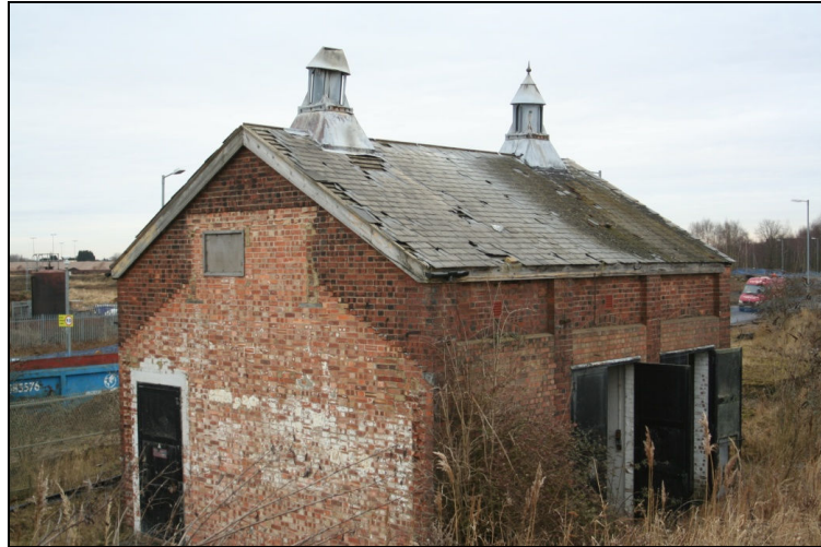
Plate 2. The Shed, showing the outline of a former extension to the building, looking northeast
