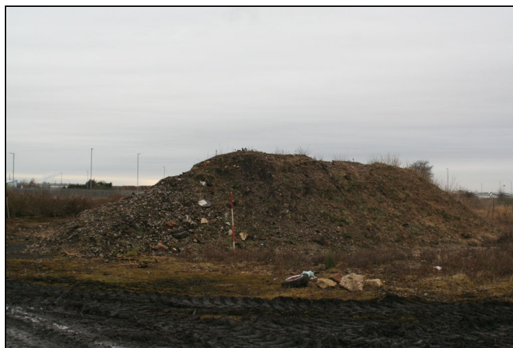
Plate 20. Air Raid Shelter #1 (Structure 21) looking southwest
