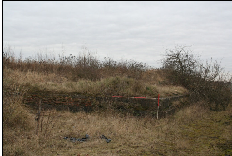
Plate 3. Structure 02 looking east.
