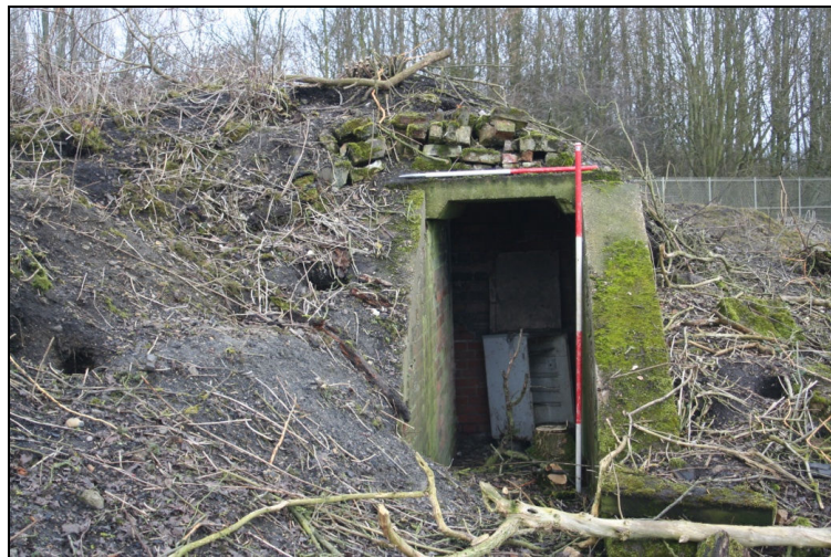
Plate 24. Entrance to Air Raid Shelter #5 (Structure 25) looking north
