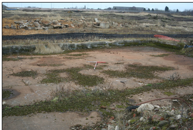
Plate 8. Water cooling tank (Structure 07) looking southeast.
