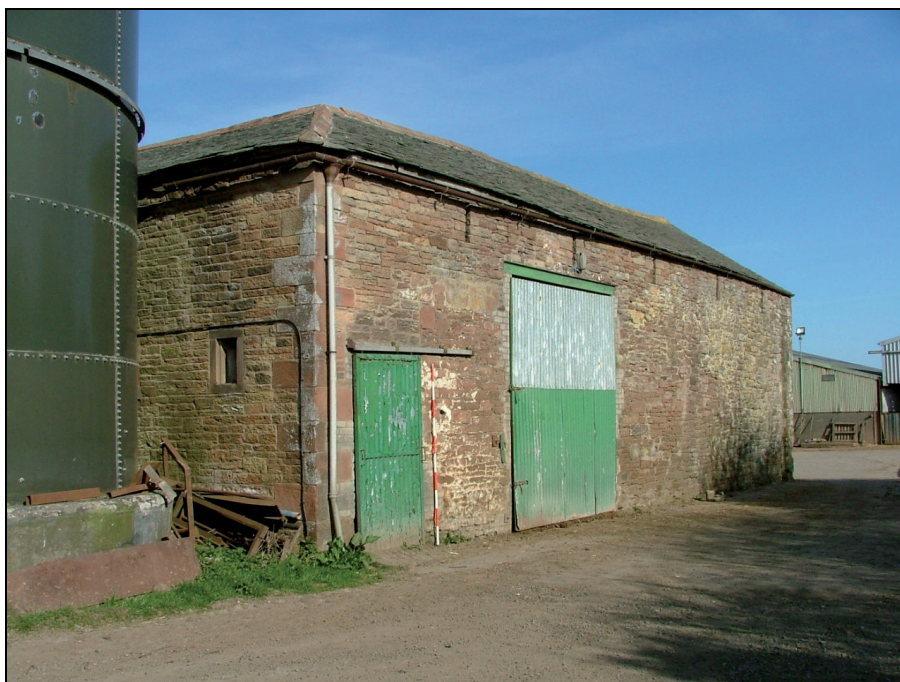
Plate 3: View looking north-west showing the east elevation (Scale = 2m)
