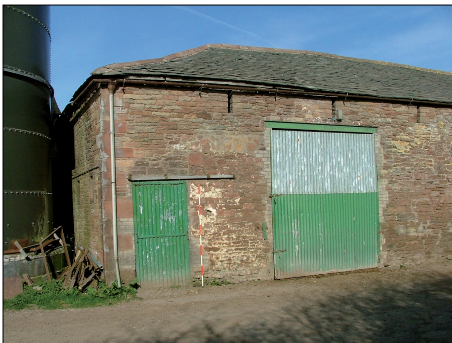
Plate 7: East elevation showing the two inserted doorways (Scale = 2m)
