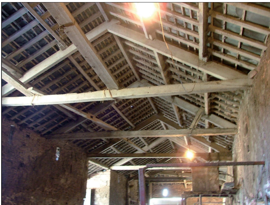
Plate 32: View looking east showing the roof structure of the barn at High Aketon Farm
