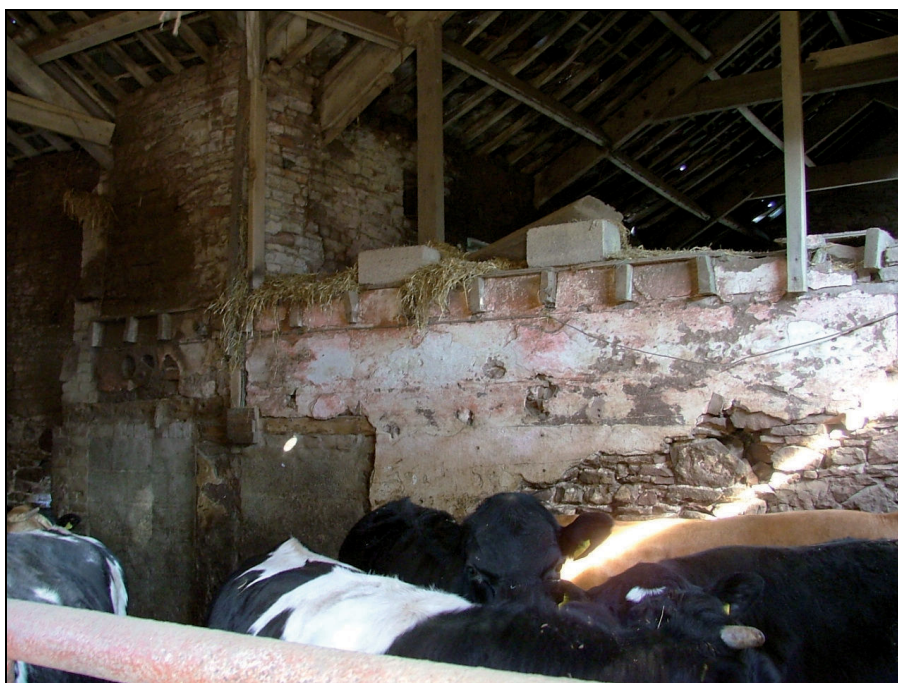
Plate 26: Masonry wall which separates the east end of the barn from the survey building at ground floor level, showing two blocked doorways to left of photograph
