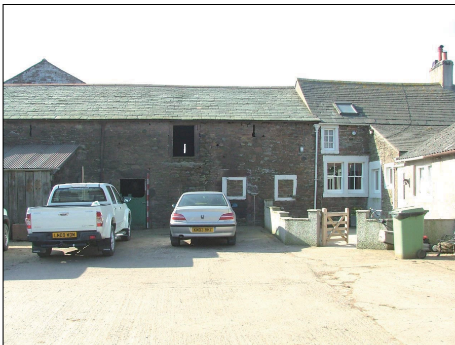
Plate 29: Western end of the barn adjoining the house, north elevation (Scale = 2m)
