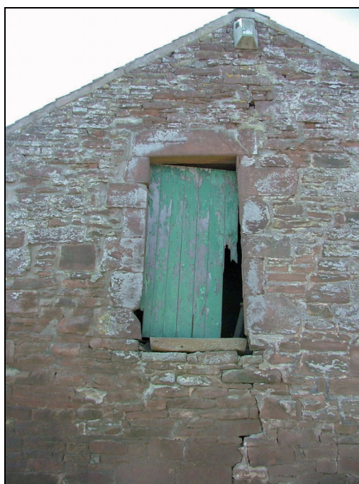
Plate 13: Detail of the first floor doorway in the north elevation
