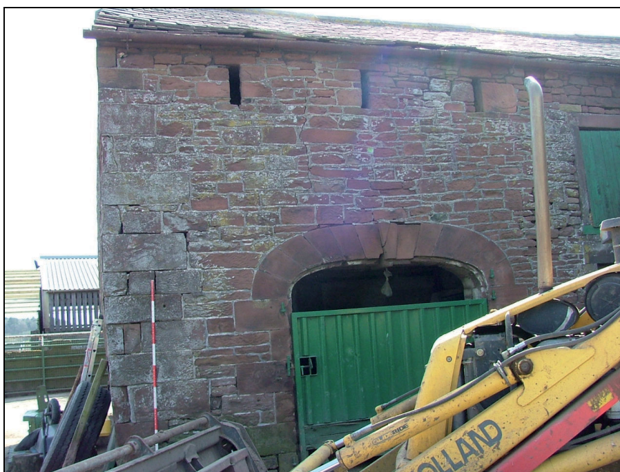
Plate 15: West elevation showing alternating quoins (Scale = 2m)
