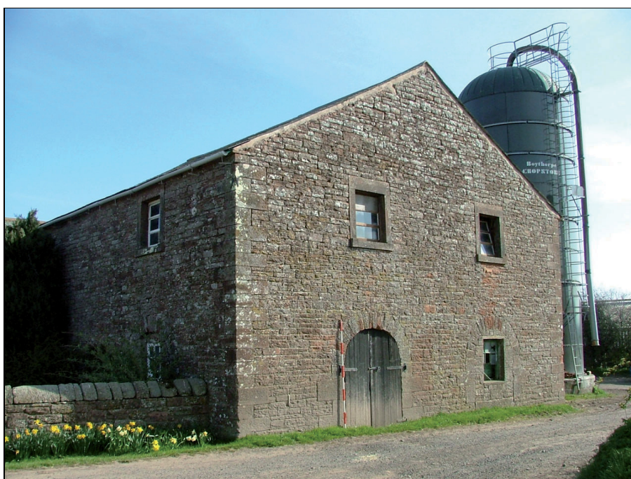
Plate 38: South elevation of Building A (Scale = 2m)
