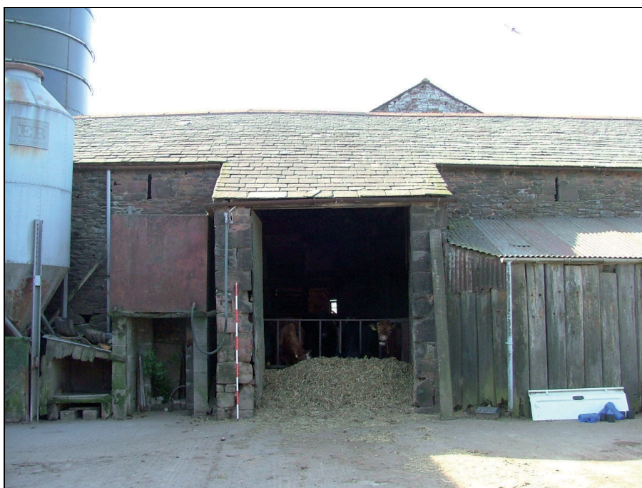
Plate 28: Main doorway into barn, north elevation (Scale = 2m)
