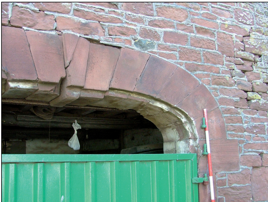
Plate 16: Detail of the voussoirs over the cart shed door, west elevation
