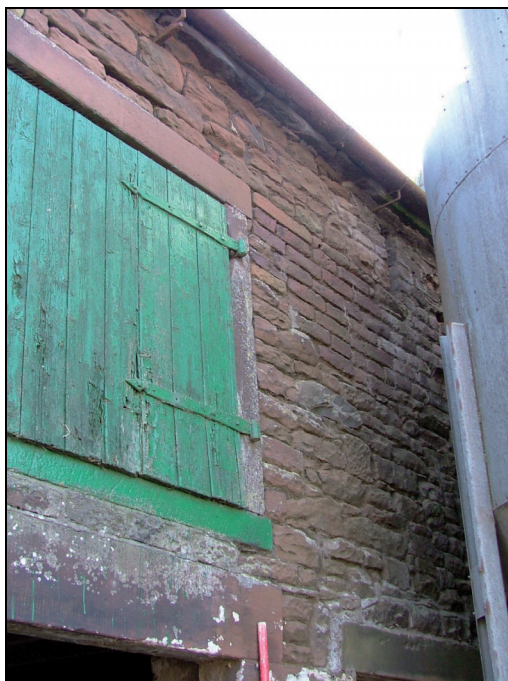
Plate 19: West elevation showing area of brickwork above the ground floor window
