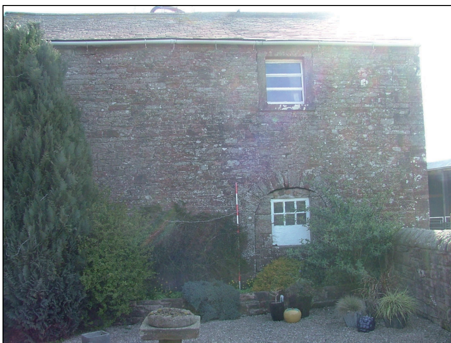
Plate 40: West elevation of Building A (Scale = 2m)
