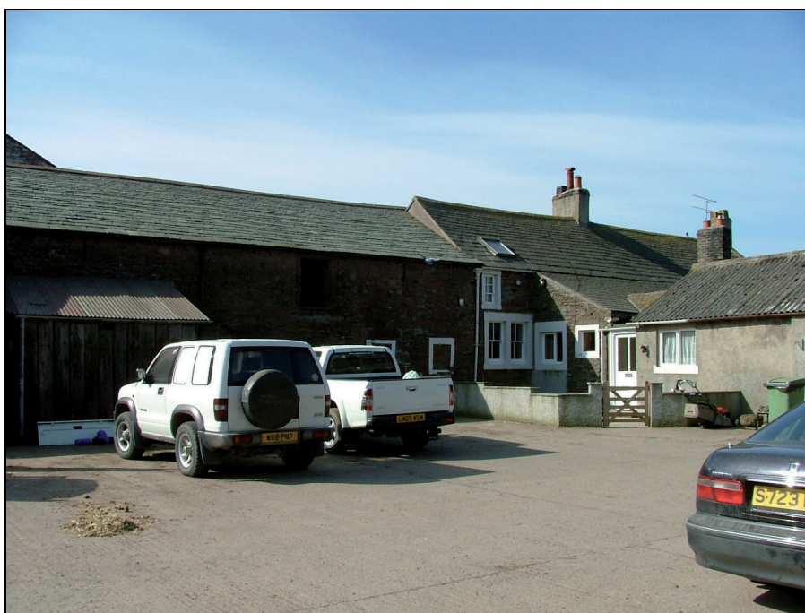
Plate 36: North elevation of the farmhouse located at the west end of the barn
