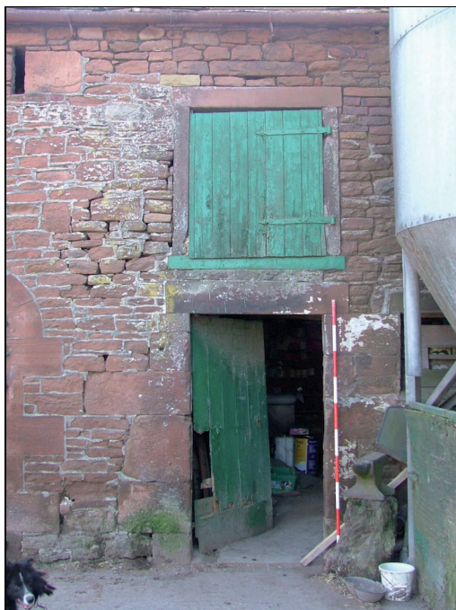
Plate 17: Doorway with pitching hole above, west elevation (Scale = 2m)
