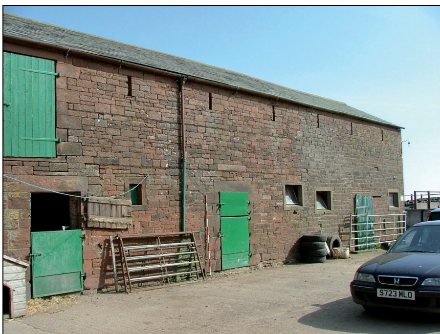
Plate 44: View looking north-east showing the south elevation of Building B
