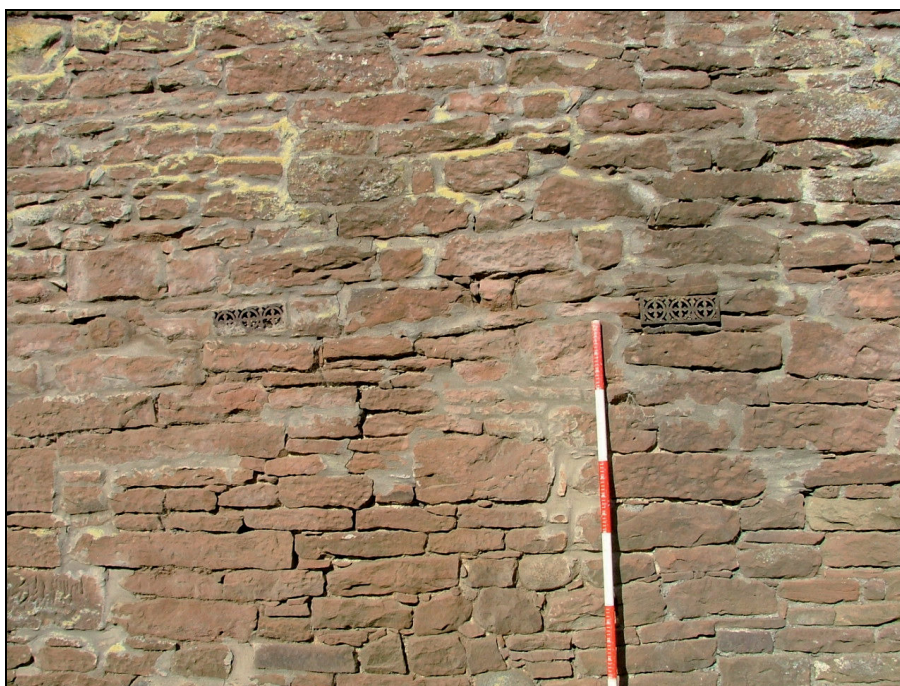
Plate 11: Detail of two cast iron decorative 'air bricks'
