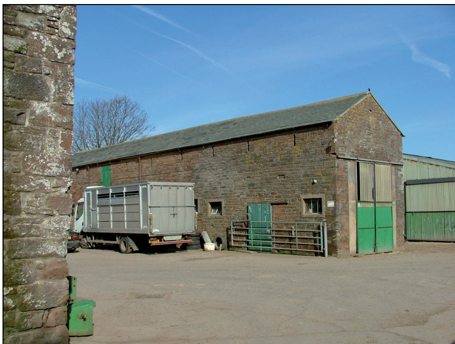
Plate 43: View looking north-west showing the east and south elevations of Building B
