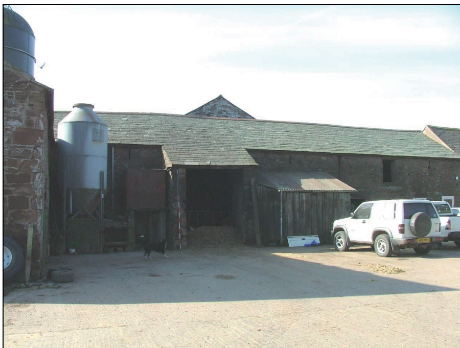
Plate 27: North elevation of the barn
