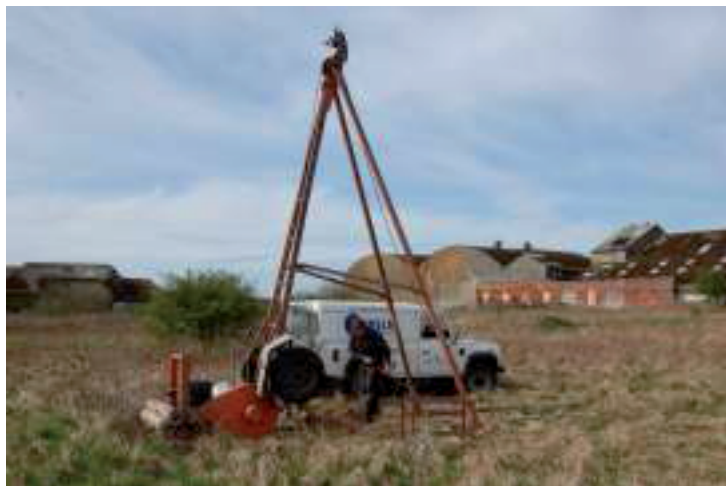
Plate 3: Mobile Bore Rig at Bore Hole #5
