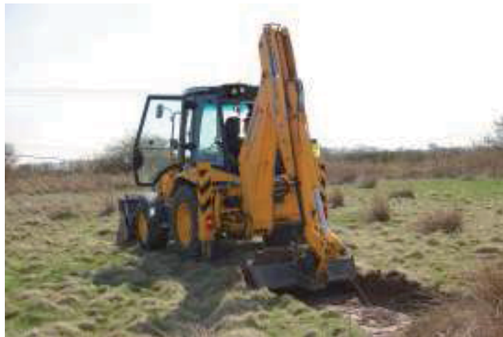
Plate 1: Mechanical Excavator Working on Test Pit #12
