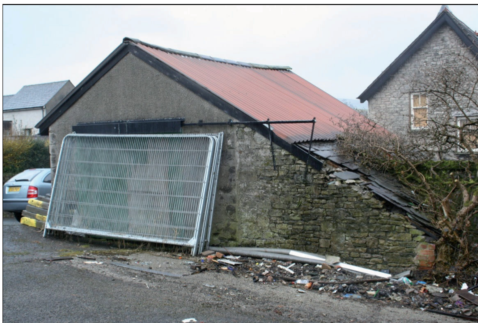
Plate 11: Rear of the former stable building and wash house, looking northeast
