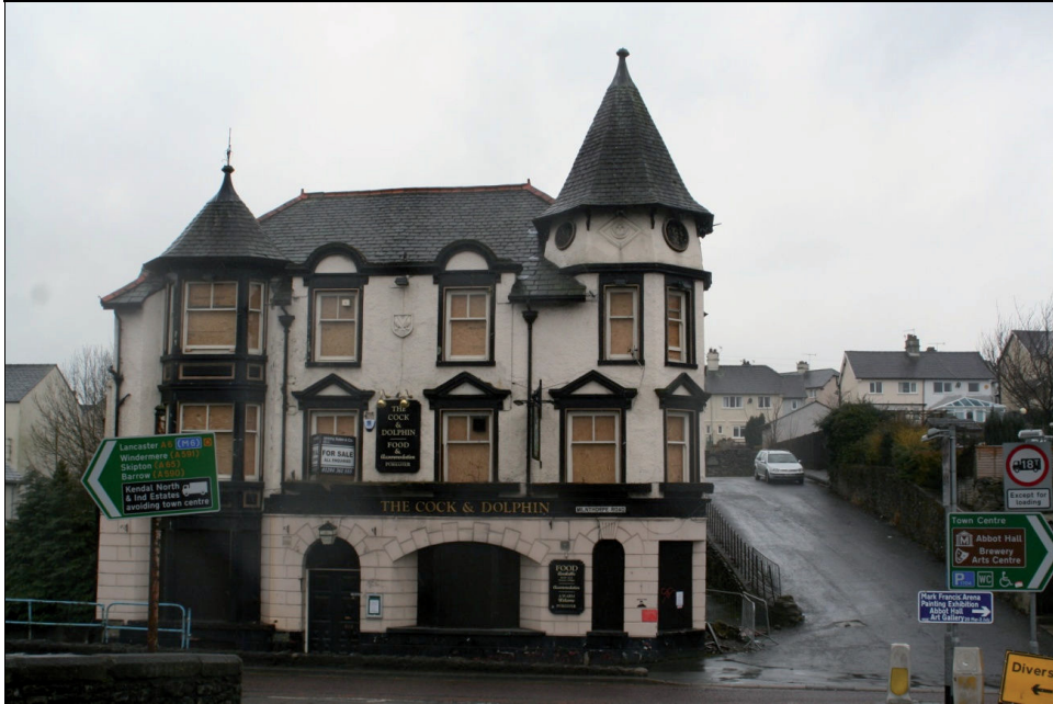
Plate 3: The vacant Cock & Dolphin Public House, looking west
