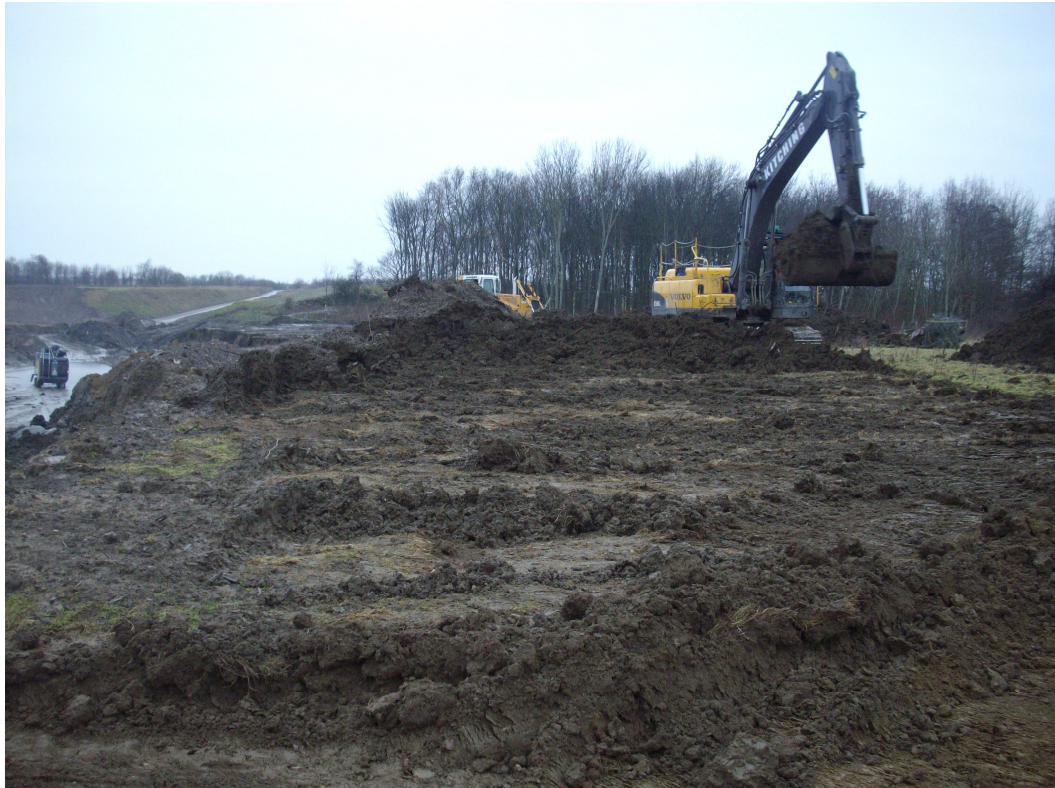
Plate 1: General shot of stripping in progress.
