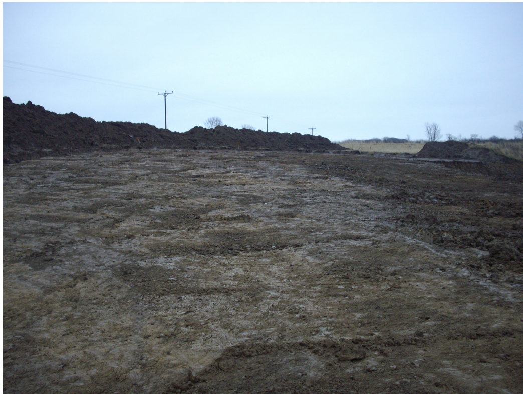
Plate 2: Stripped Area, looking west.
