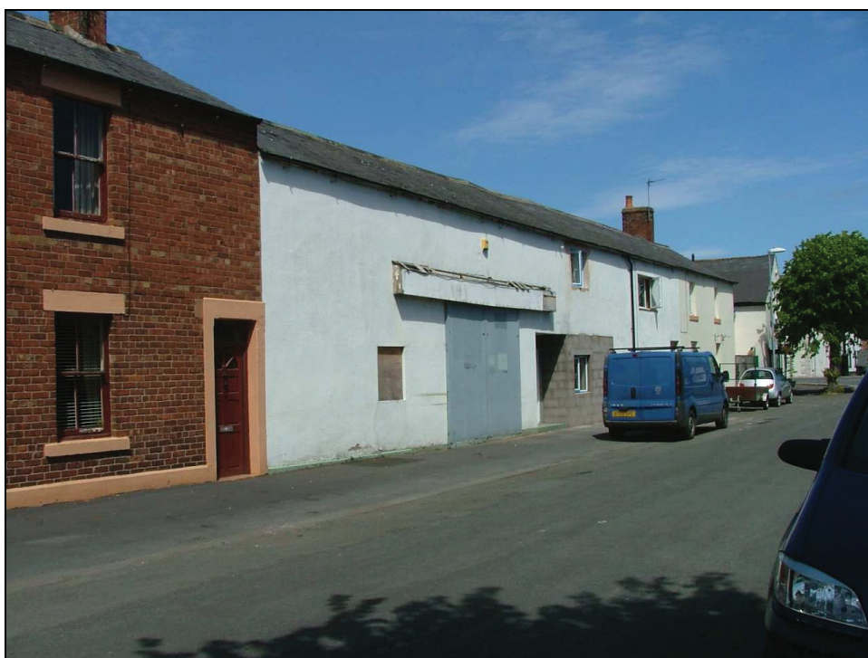
Plate 2: The former Greenalls Garage on the north side of Bank Street
