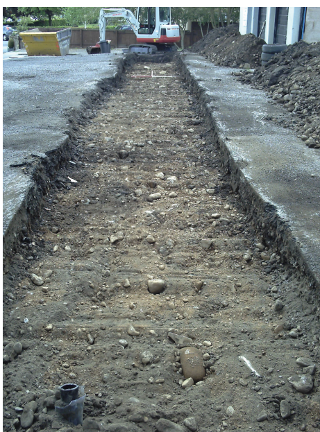
Plate 11: Trench 1 general view looking south
