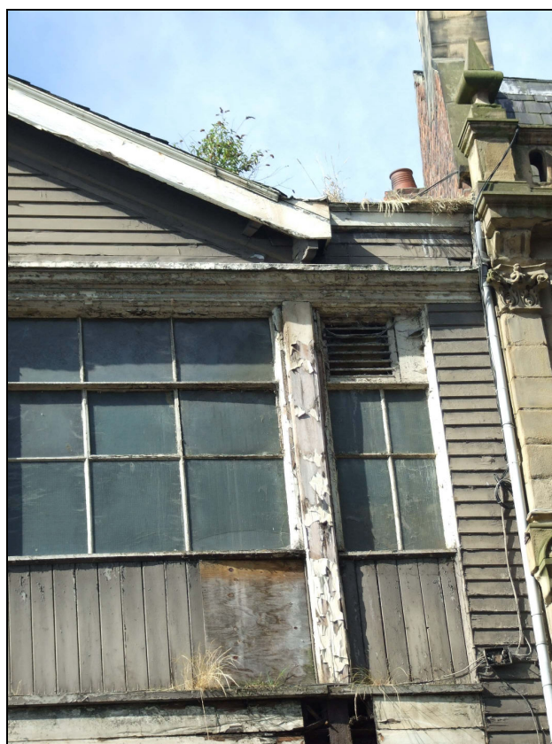
Plate 3: Smaller window and vent at northwestern aspect of Westgate Road frontage
