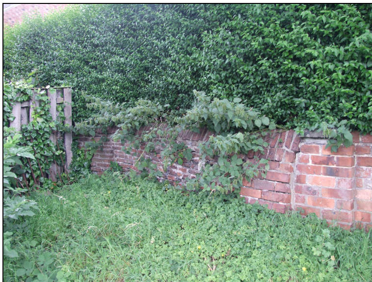
Plate 11: Brick boundary wall between the grave markers and Bellevue Bungalow, note the older brickwork
