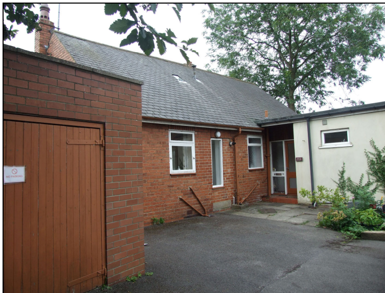
Plate 4: Northern elevation of Bellevue Bungalow, note the more modern extension
