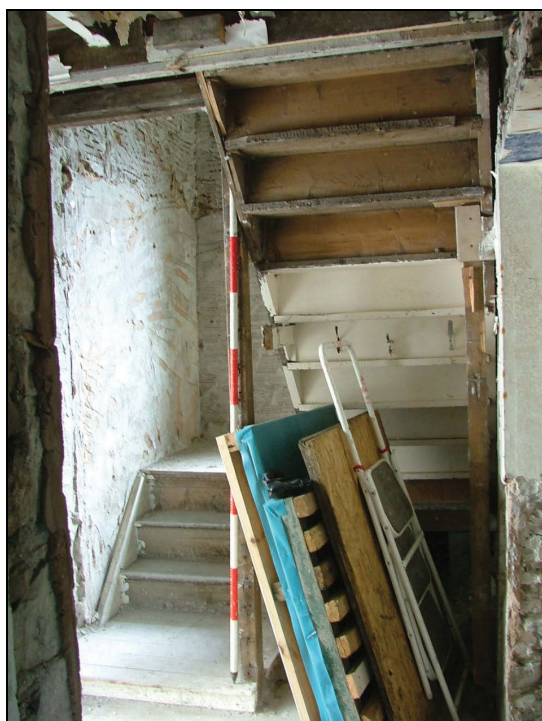
Plate 46: Staircase as seen from the ground floor
