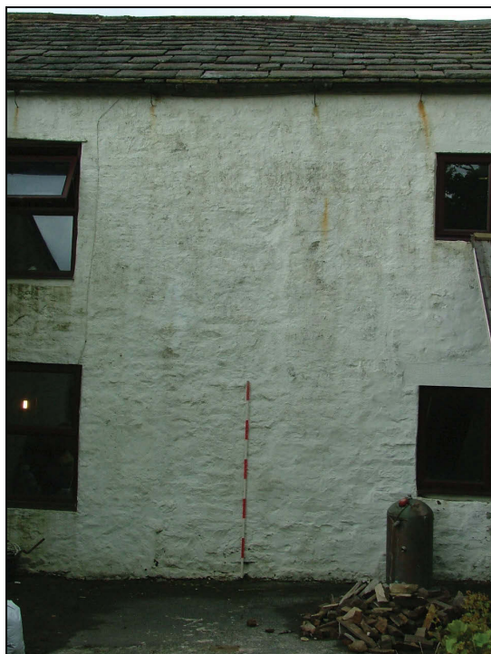
Plate 14: Possible vertical construction break in the south-east elevation or former doorway (Scale = 2m)
