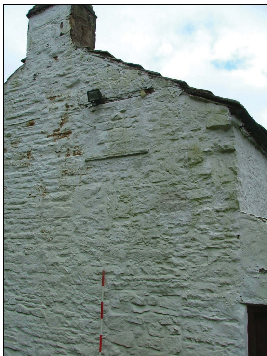
Plate 11: North-east elevation showing blocked window
