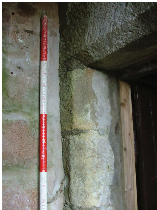
Plate 24: Detail of the chamfer in the door surround, south-west elevation
