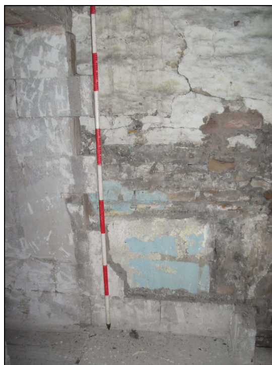
Plate 68: Blocked window in the north-west wall of Bedroom 2
