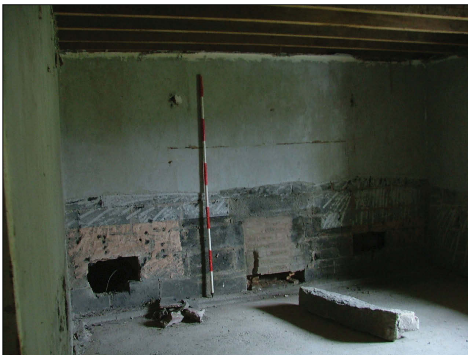
Plate 41: North-east wall of Reception Room 2 showing the blocked-up fireplace (Scale = 2m)
