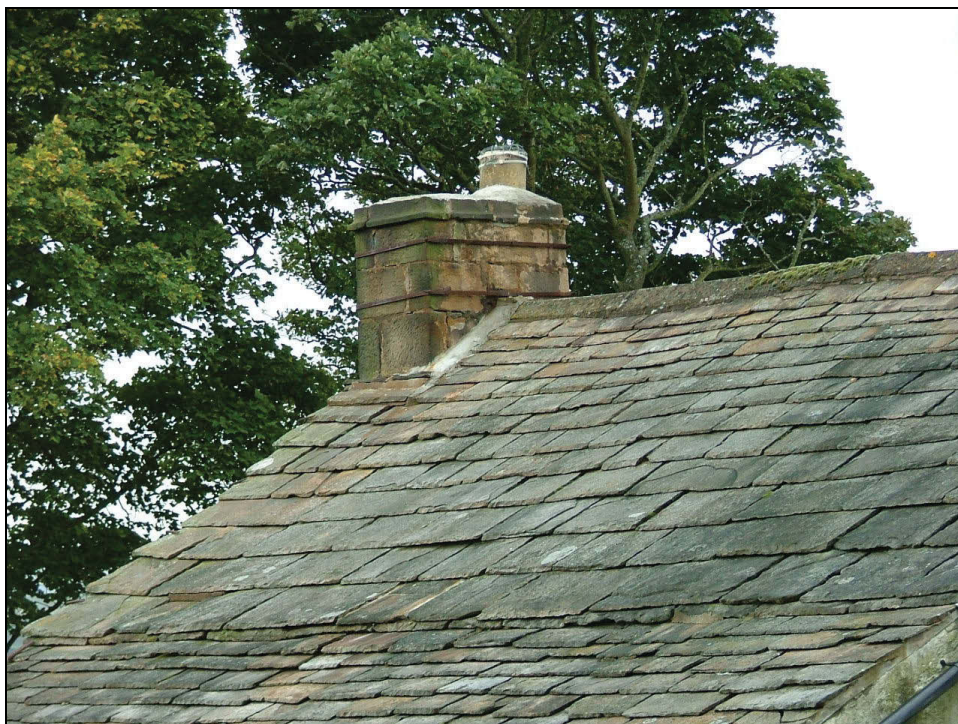
Plate 26: Detail of the chimney stack, south-west end of the house
