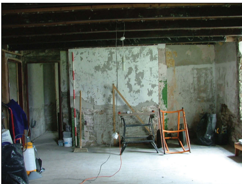
Plate 40: View looking north-east showing possible former range in Reception 1 (Scale = 2m)
