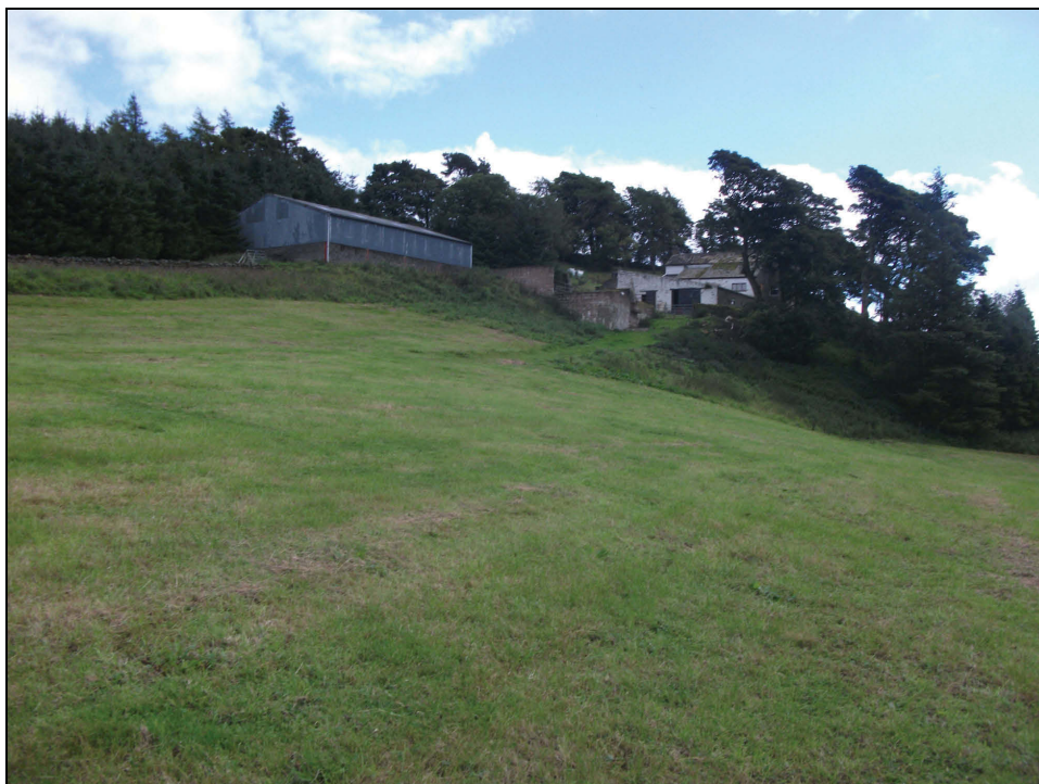
Plate 6: View looking south-east showing the farm buildings to the north-west side of the house at High Scilly Hall
