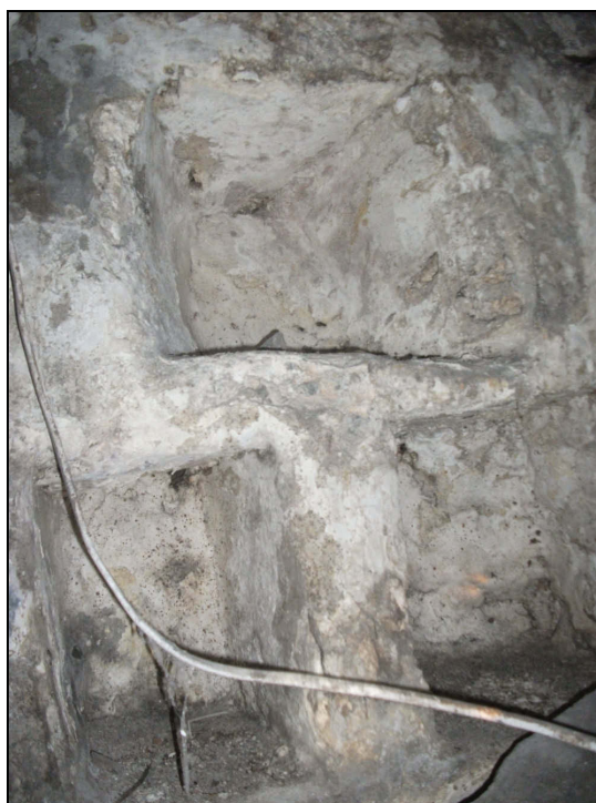
Plate 42: Detail of hidden 'shelves' within the north-west wall of Reception Room 2
