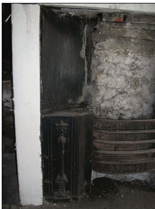
Plate 56: Detail of the decoration on the fire grate, Bedroom 1
