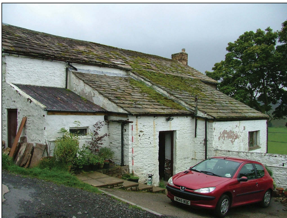
Plate 27: Detail of the three outshuts against the north-west elevation of the main house (Scale = 2m)
