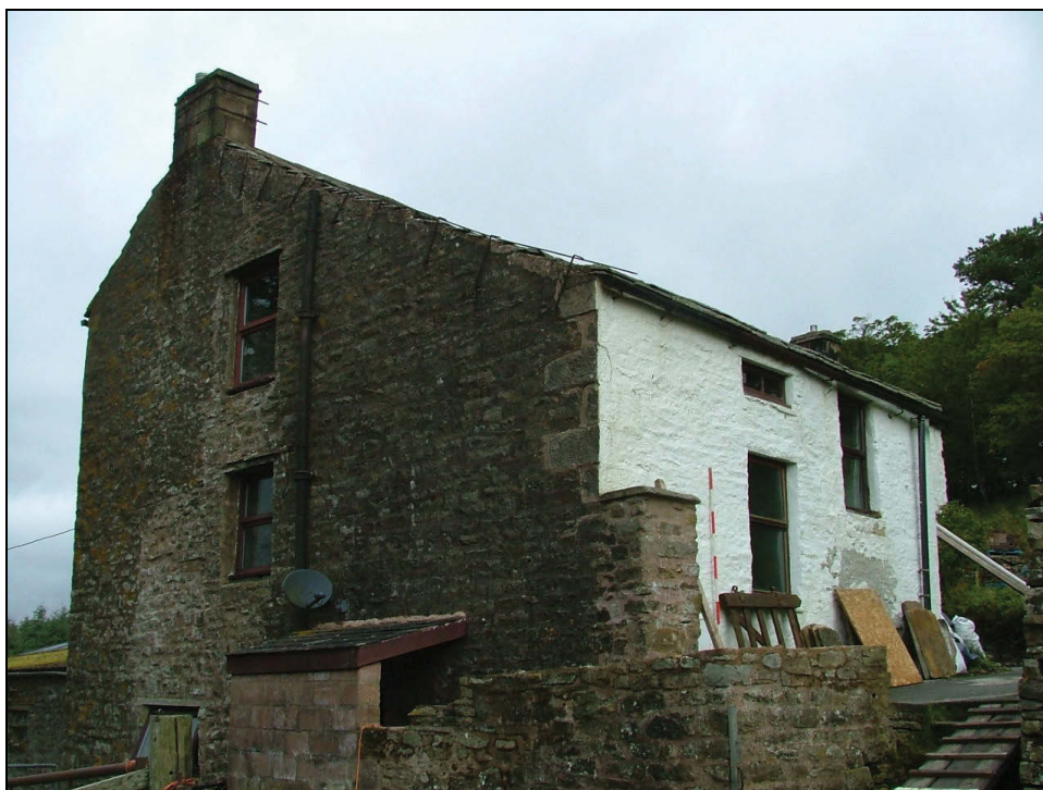
Plate 21: View looking north showing the south-west elevation of High Scilly Hall
