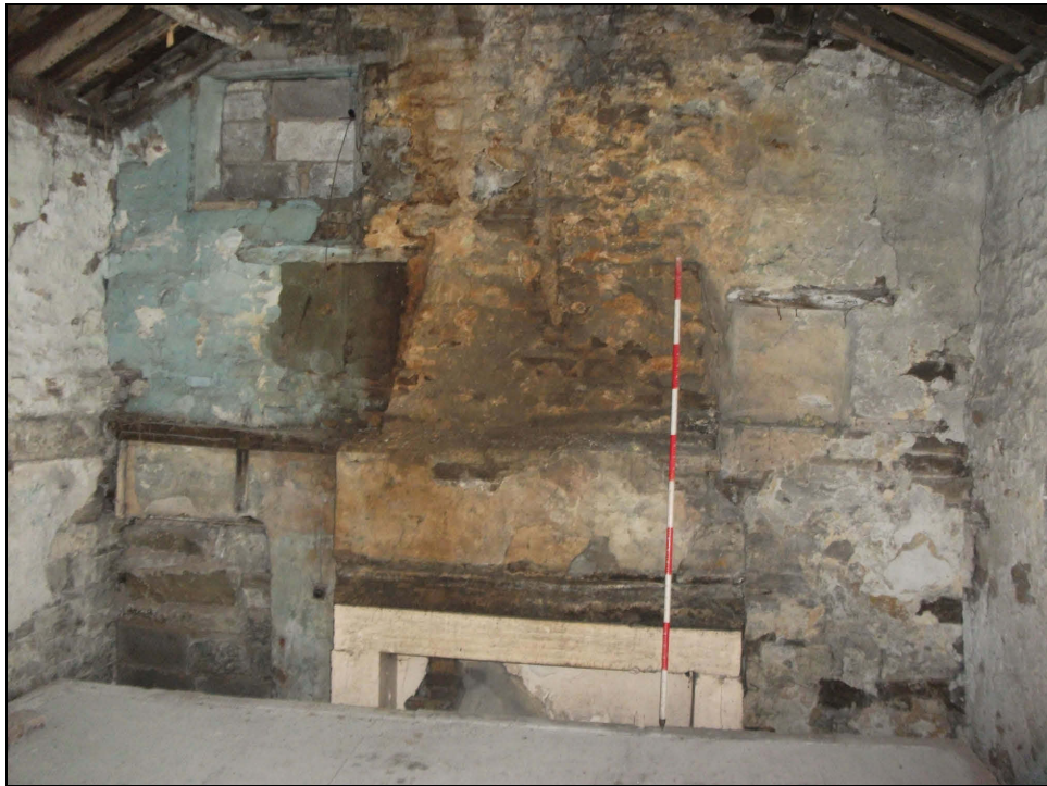
Plate 61: North-east elevation of Bedroom 2 showing the top of a former fireplace, change in floor level and blocked up windows (Scale = 2m)
