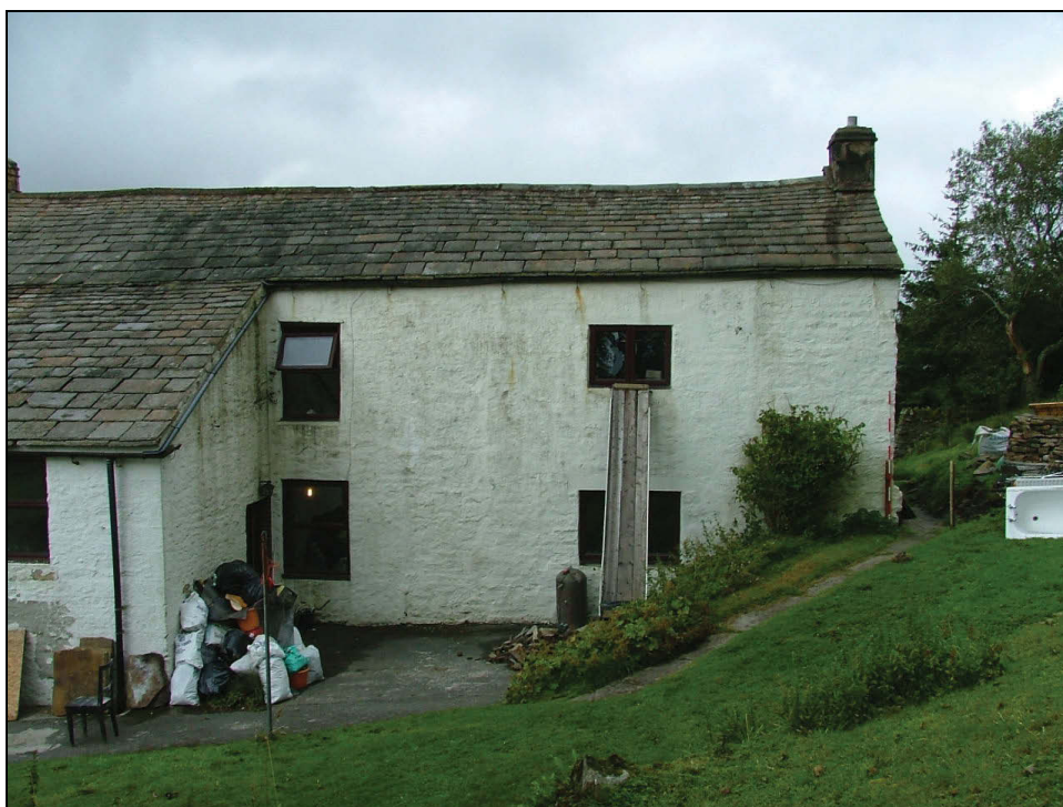
Plate 13: North end of the south-east elevation
