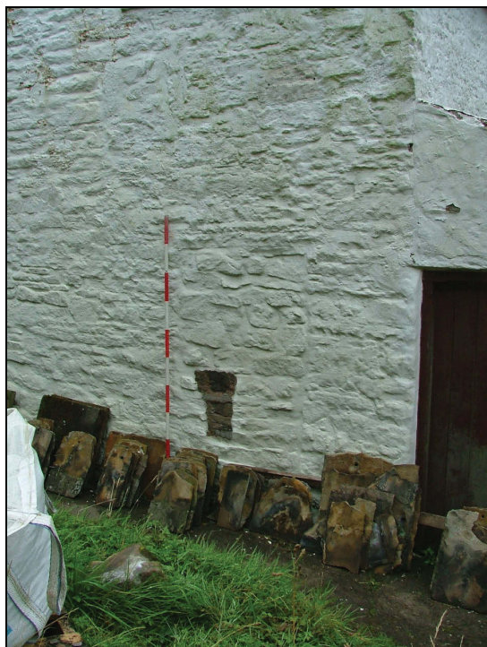
Plate 10: Blocked doorway, north-east elevation (Scale = 2m)
