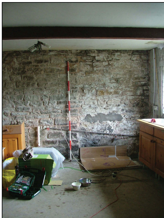
Plate 35: Blocked window in the south-west wall of the kitchen (Scale = 2m)
