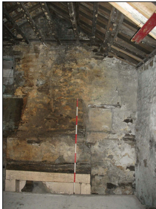
Plate 62: Blocked window to the right of the fireplace, Bedroom 2 (Scale = 2m)
