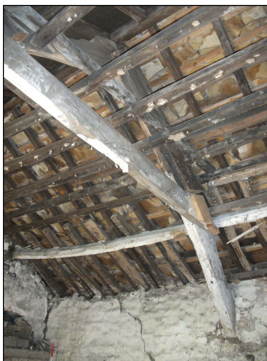
Plate 58: Detail of the roof truss over Bedroom 2
