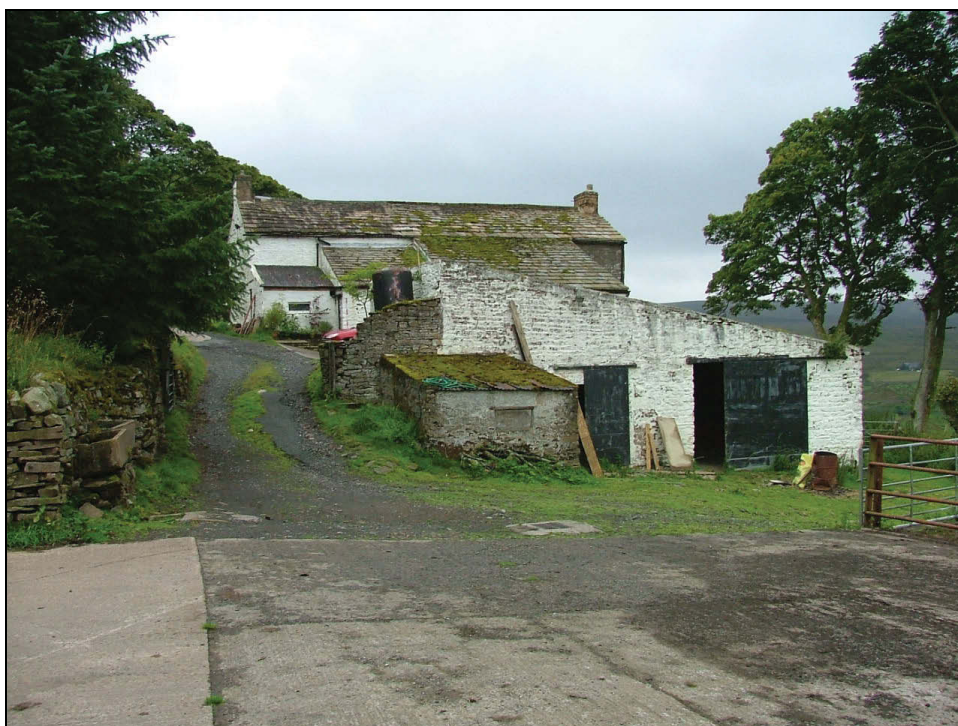
Plate 32: View looking south-east showing the stone-built farm buildings to the north-west side of the house
