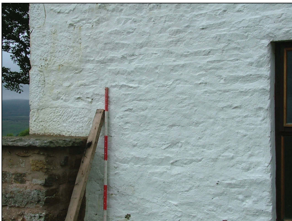
Plate 19: Possible blocked window, south-east elevation of outshut
