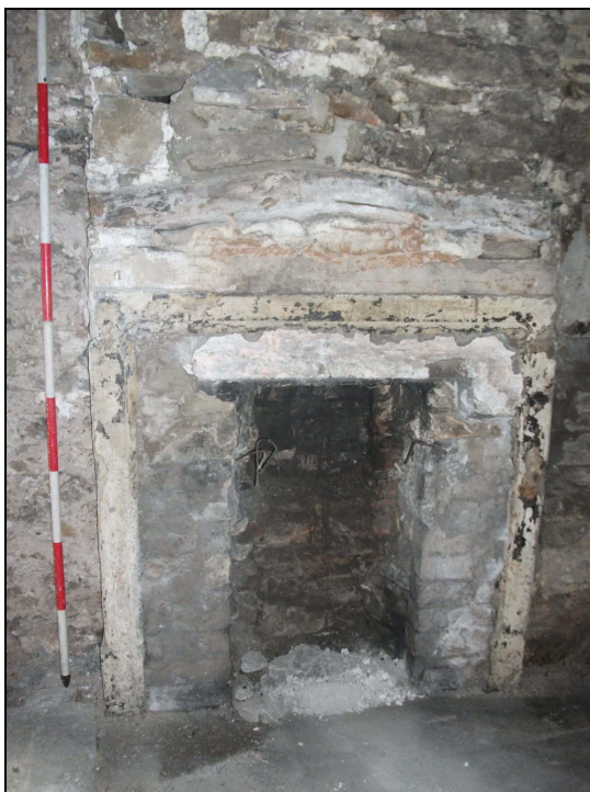
Plate 51: Detail of the fireplace in Bedroom 1
