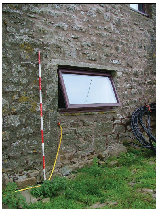
Plate 25: Modern window inserted into a former doorway, south-west elevation (Scale = 2m)
