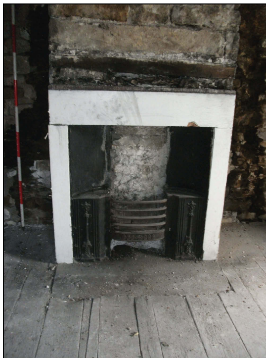
Plate 55: Detail of the fireplace in the north-east wall of Bedroom 1
