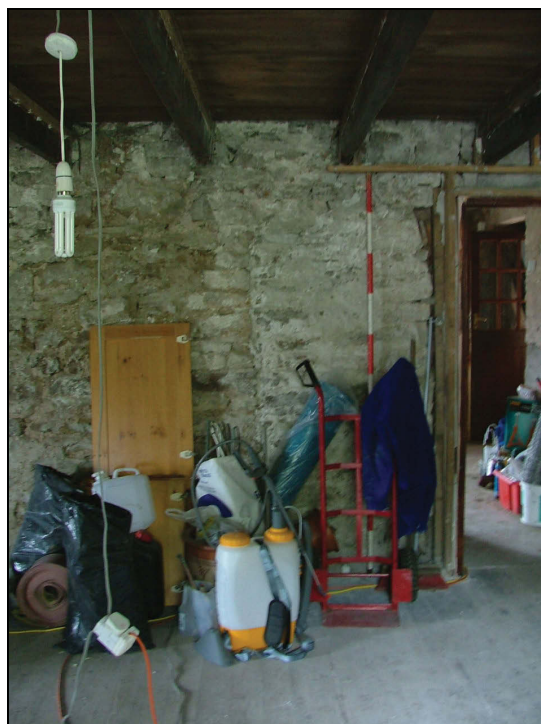
Plate 38: Possible former doorway, north-west wall of Reception Room 1 (Scale = 2m)
