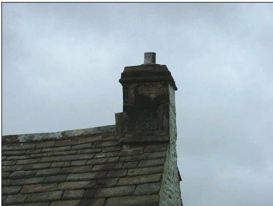
Plate 12: Detail of the chimney stack, north-east elevation
