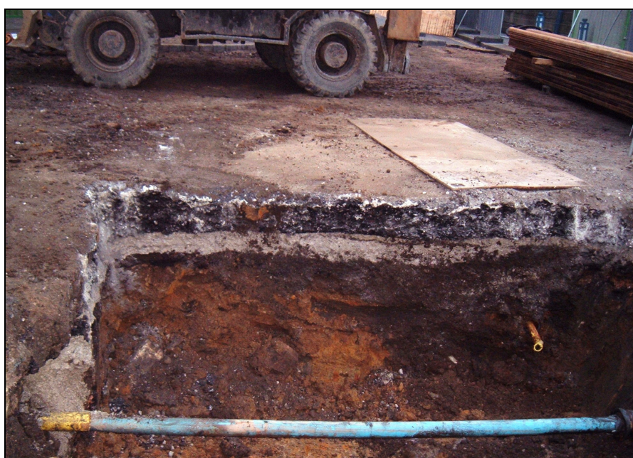
Plate 7: West facing section within Trench 3, showing cut for service trench [303]
