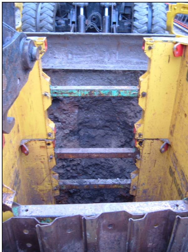
Plate 3: East facing section through deposits in Trench 1.
