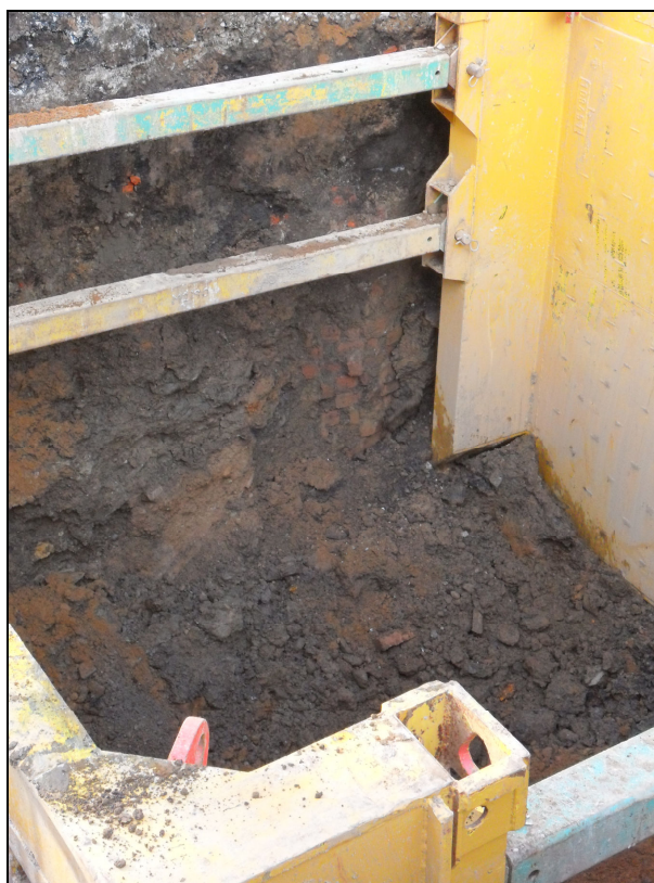
Plate 8: South facing section of Trench 4, showing coursed brick from manhole (403)
