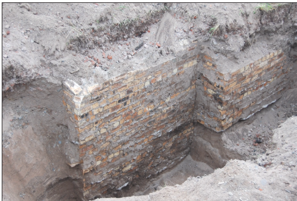
Plate 2: Northeast elevation of wall (113)
