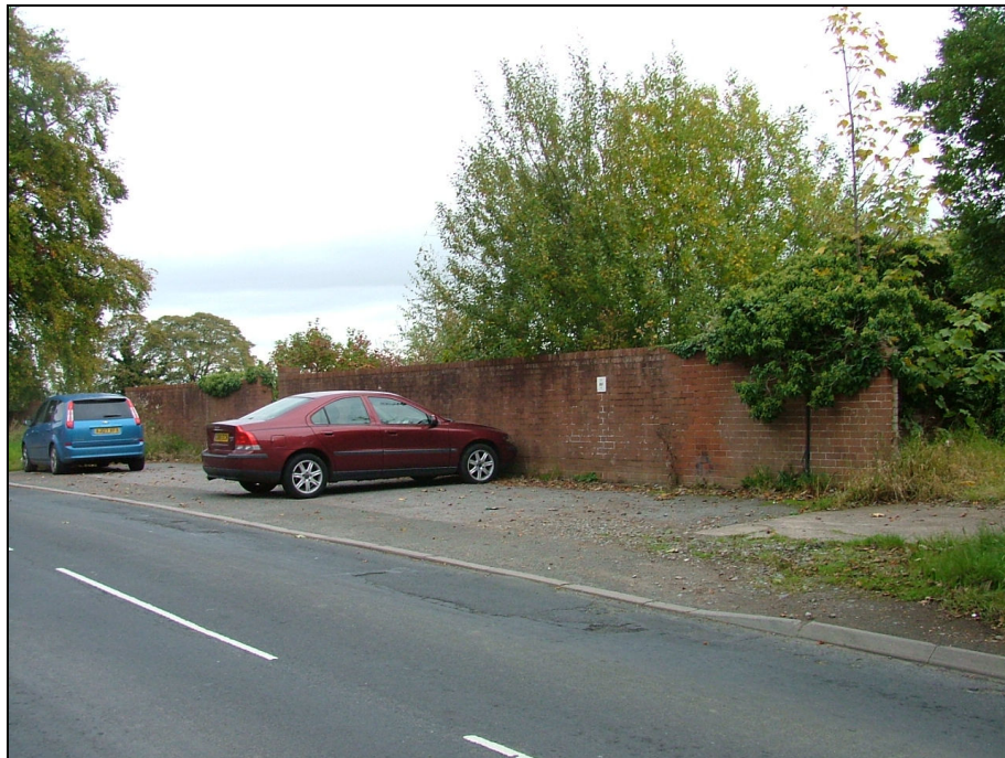
Plate 6: Brick wall along Scotby Road
