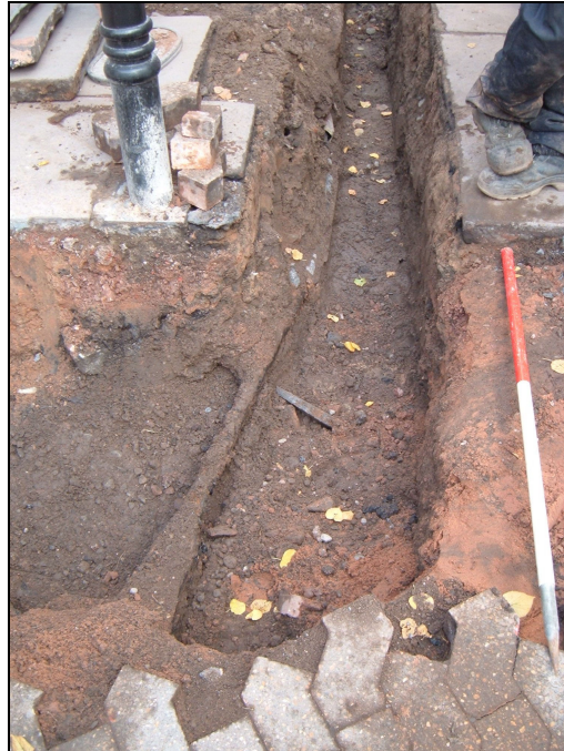
Plate 11: Located outside the 18-24 Scotch Street, just visible is a small section of tram track at the base of the trench facing east
