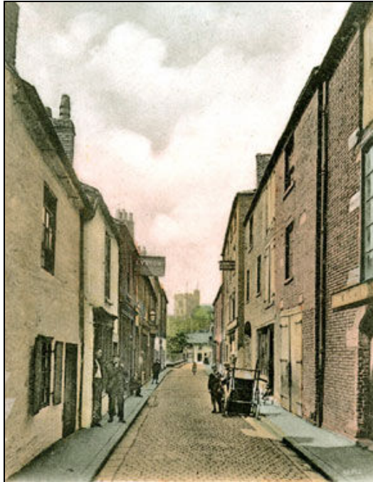
Plate 5: View looking north from the southern end of Blackfriars Street in 1905 showing buildings on the left which have now gone (Courtesy of Carlisle Library)
