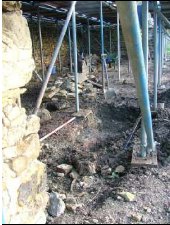
Plate 6: View looking east showing the location of Hole 3
