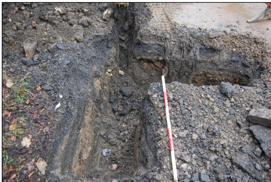
Plate 2: Trench to the rear of Hexham Road, Throckley, looking east
