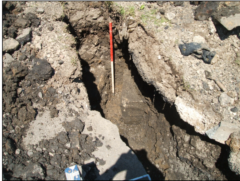
Plate 3: View of limestone block (124), Hexham Road, Throckley, looking north
