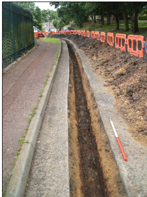
Plate 6: Trench within West Denton Road, Denton Burn, looking east
