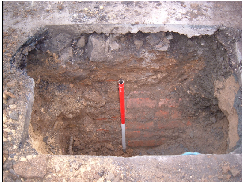
Plate 5: Trial-hole showing culvert (136) between Burt and Beverley Terraces, Walbottle, looking south
