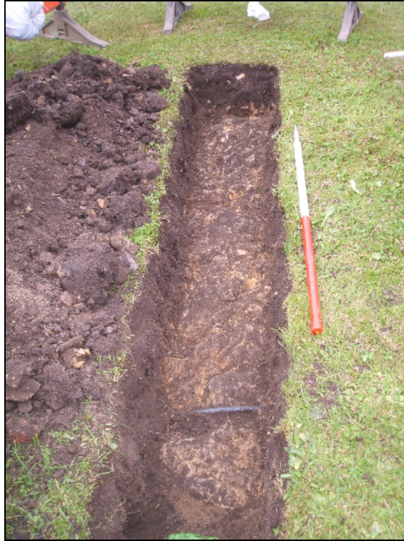
Plate 7: Foundations (115) within centre of excavated area, Avalon Drive, Denton Burn, looking east-southeast
