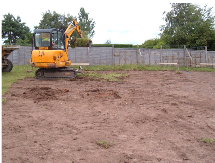
Plate 1: The excavation of the stable block platform, looking north east.
