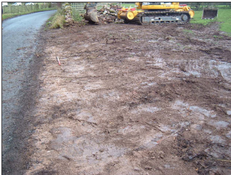
Plate 1: View northwest of Trench 1
