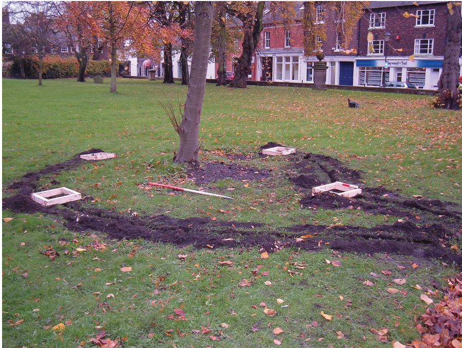
Plate 2: Tree six showing cable and light trenches facing west.
