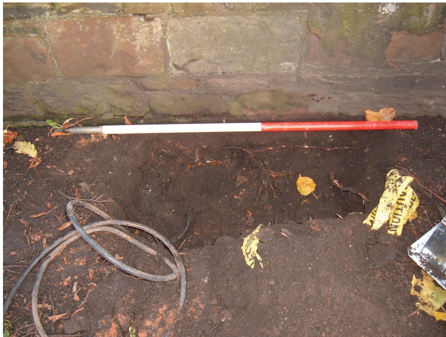
Plate 1: Foundation trench for electrical junction boxes Carlisle Cathedral Precinct.
