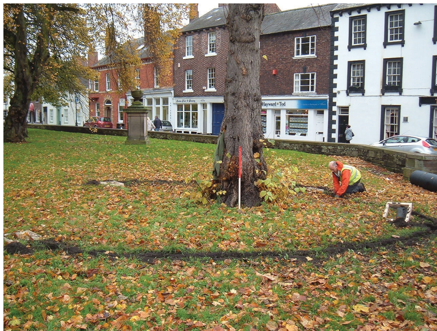
Plate 3: Tree seven showing cable and light trenches facing west.
