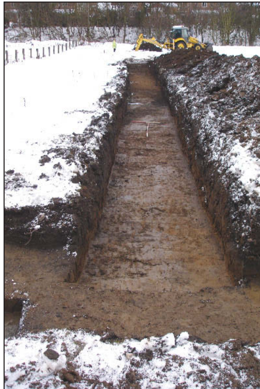
Plate 8: Trench 8 looking southeast
