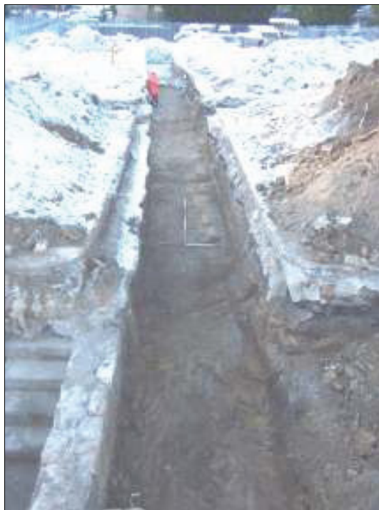
Plate 1: Trench 1 (looking west-southwest)
