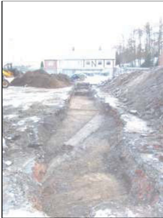
Plate 3: Trench 2 after cleaning (looking south-south west)
