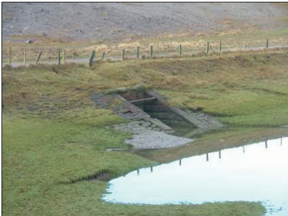
Plate 14: Detail of the masonry outfall located to the north side of the proposed pipeline in Section 1 of the walkover route
