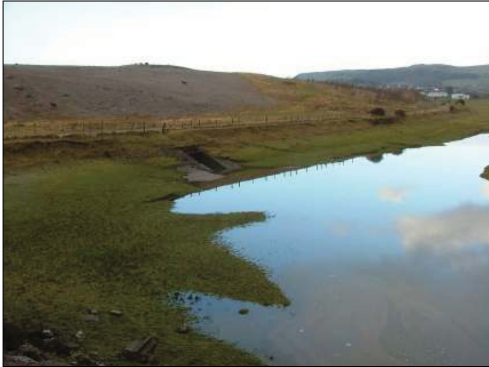
Plate 13: View looking west from the top of the levelled slag heap showing a well-built masonry outfall located to the north side of the proposed pipeline route
