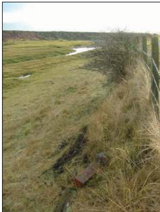
Plate 10: View looking south-east showing some brickwork and demolition material in the slope to the north side of the pipeline route
