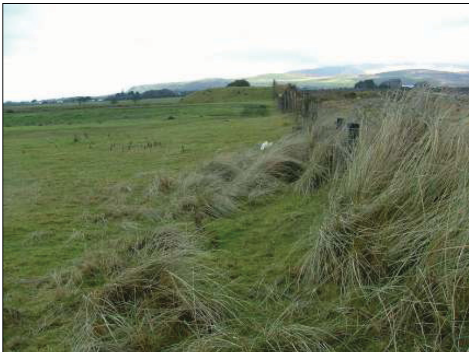
Plate 25: View looking north-west showing the easterly section of the pipeline route, Section 3 of the walkover
