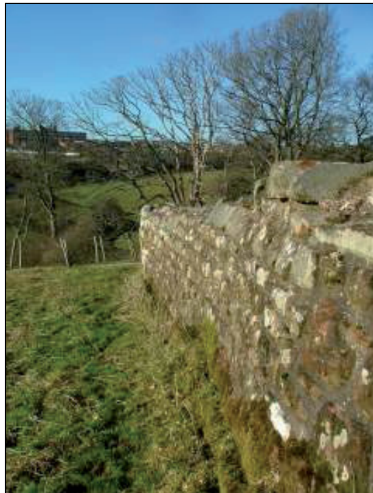
Plate 14: View looking north-east showing the section of Park Wall which serves as the north-eastern boundary of the proposed development area, with Furness General Hospital visible in the background
