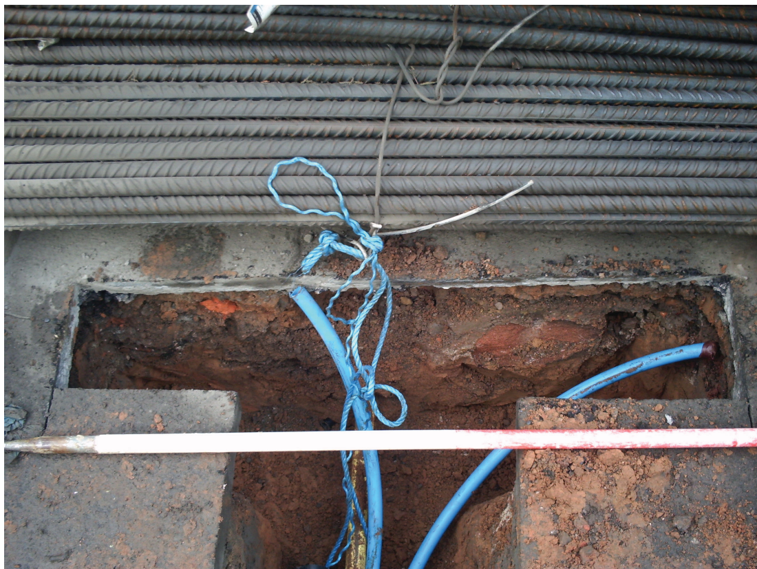
Plate 5: Shot of Trench 6, looking NW (bit of Trench 1 in the foreground)
