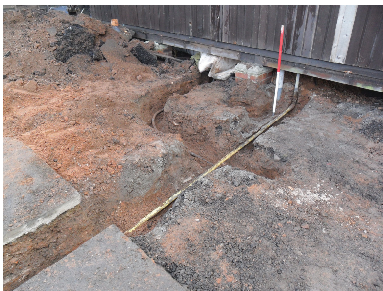
Plate 1: Shot of Trenches 1 (foreground) & 2 (background), looking E
