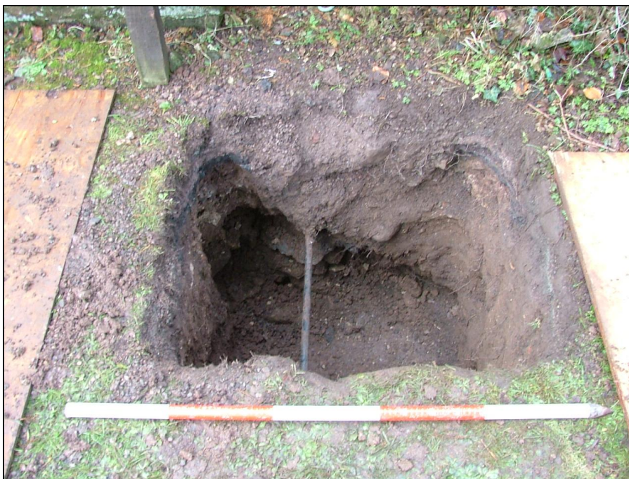
Plate 14: View looking south showing a water pipe within the pump chamber hole (Scale = 1m)
