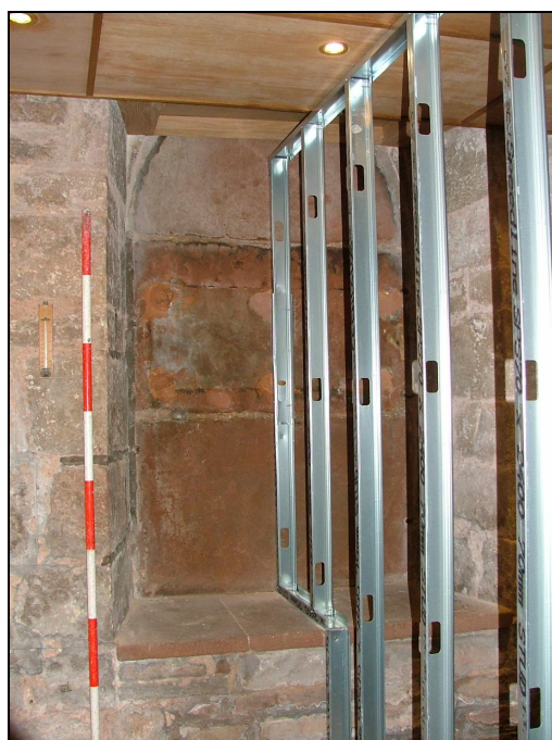
Plate 34: Internal side of the blocked
