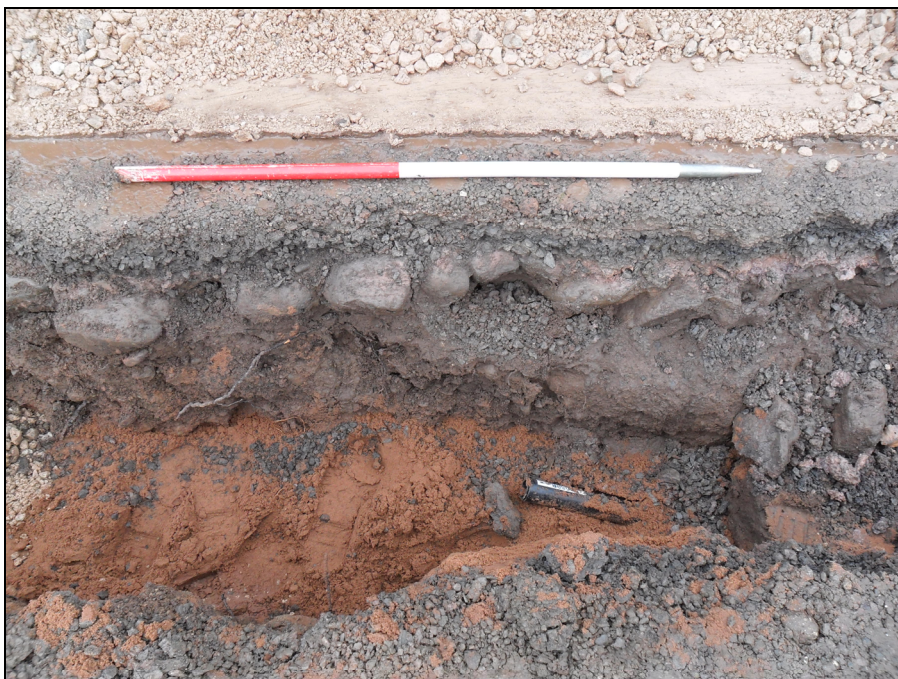
Plate 24: Detailed of possible cobbled surface located beneath the modern road to the west of the church
