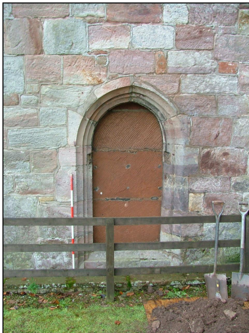
Plate 31: Blocked doorway in the north wall of the church
