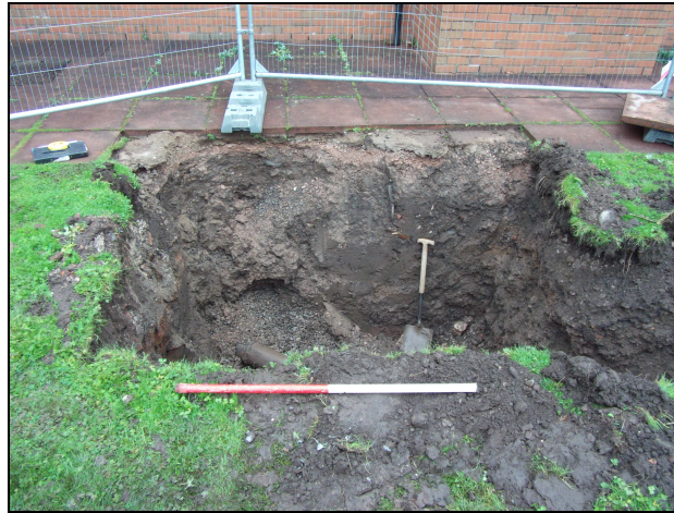
Plate 7: Excavation of Pit in Zone 3 for Two Inspection Chambers (facing north)
