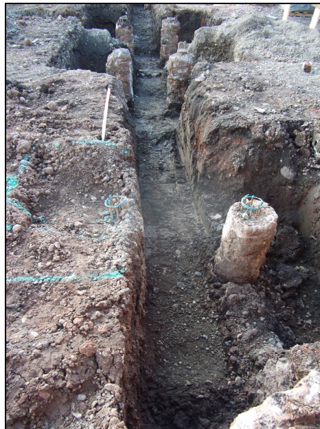
Plate 8: Foundation Trench for the New Main Building (facing north)
