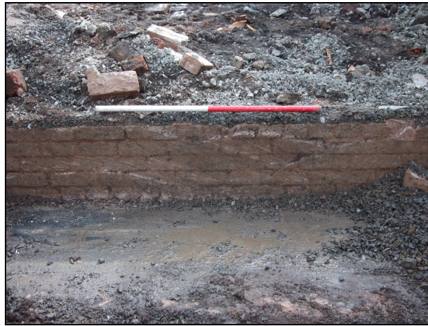
Plate 5: Redbrick Wall (108) set on Hardcore Layer (109) (facing east)
