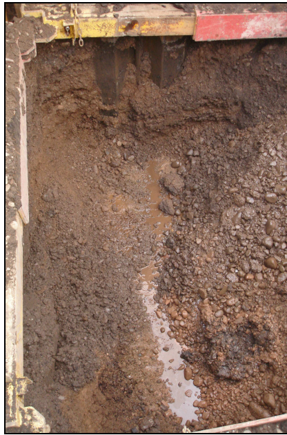
Plate 4: Natural River Gravels (128) at a depth of c.4.00m (facing east)
