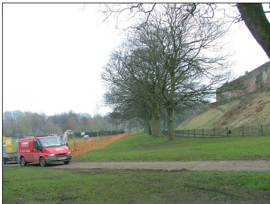
Plate 1: View looking east showing the proposed footpath route defined by the orange fencing. The north wall of Carlisle Castle is visible to the right of photograph
