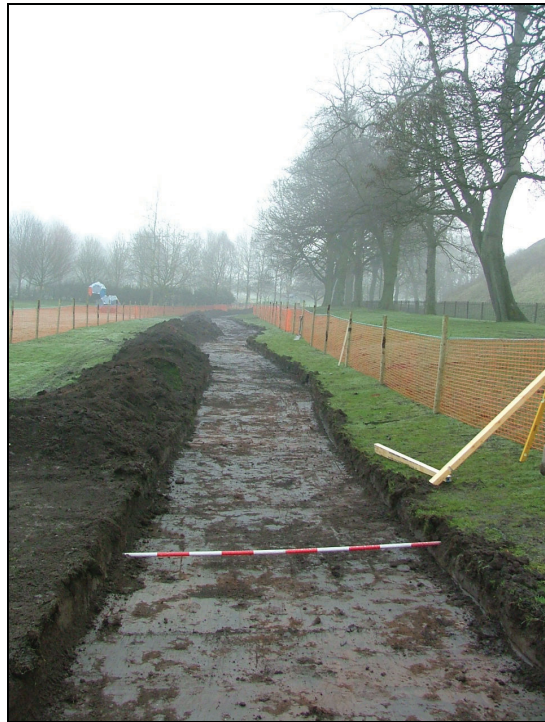
Plate 4: View looking west showing the excavated trench (Scale = 2m)
