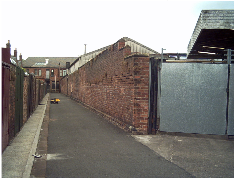
Plate 2: Western range of Ancillary building with South west corner of main northern block in background (Taken from alley running to the rear or Richardson Street)
