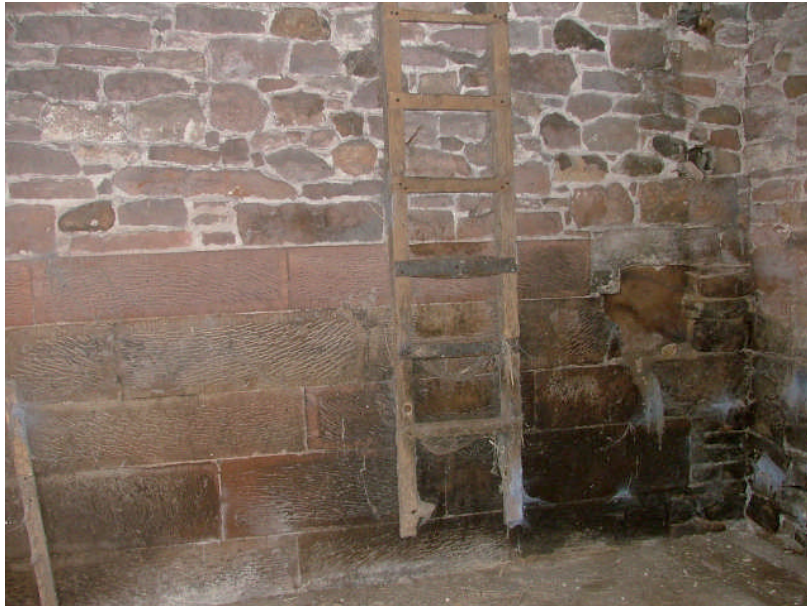
Plate 13 – Stable, dressed masonry blocks in north wall
