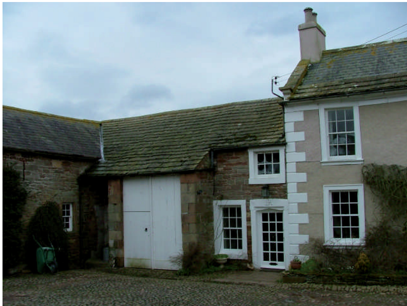
Plate 2 – East facing elevation of Barn A, showing sandstone tiled roof
