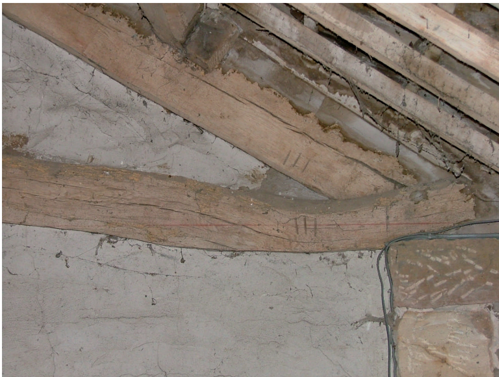
Plate 7 – Assembly marks in roof truss set into wall that divides the barn from the southern end of the house
