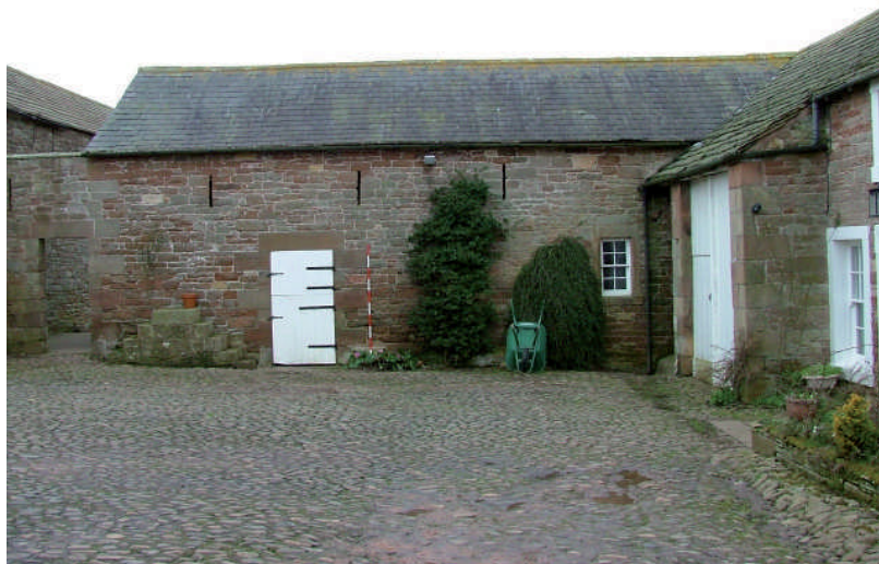
Plate 4 – North facing elevation of Barn A showing doorway to byre
