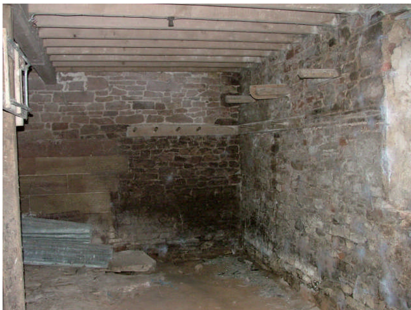
Plate 12 – Interior of stable, Barn B
