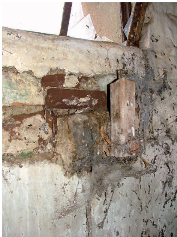
Plate 10 – Projecting stone blocks with wood attached, byres Barn B
