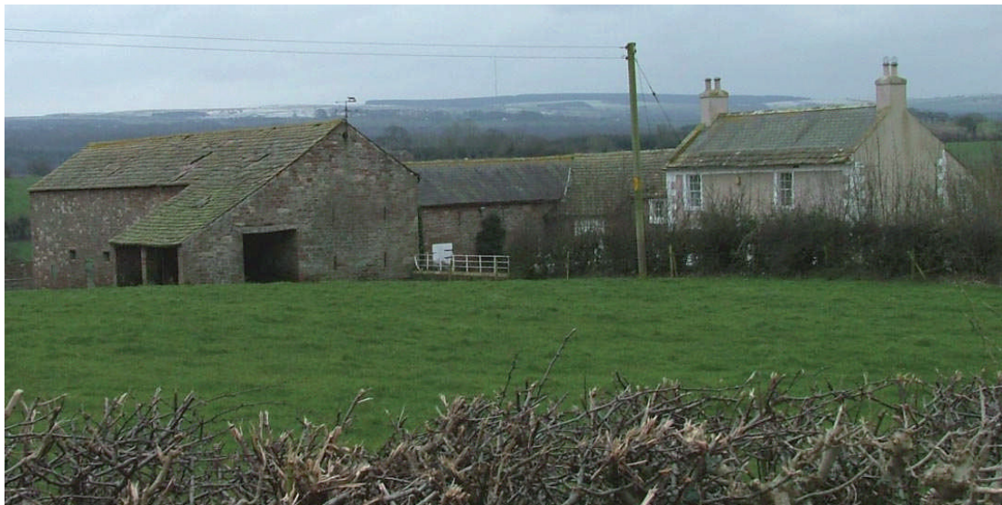
Plate 1 – Brackenthwaite Farm as seen from the road, looking south
