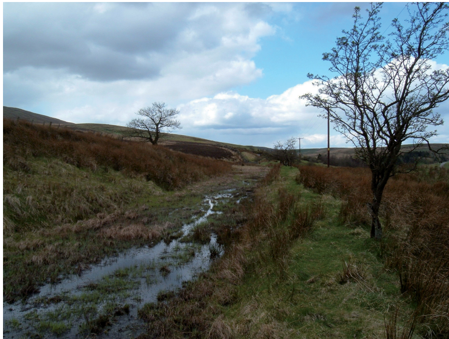
Plate 6: Wet conditions on the trackbed west of Prior High Side Drift
