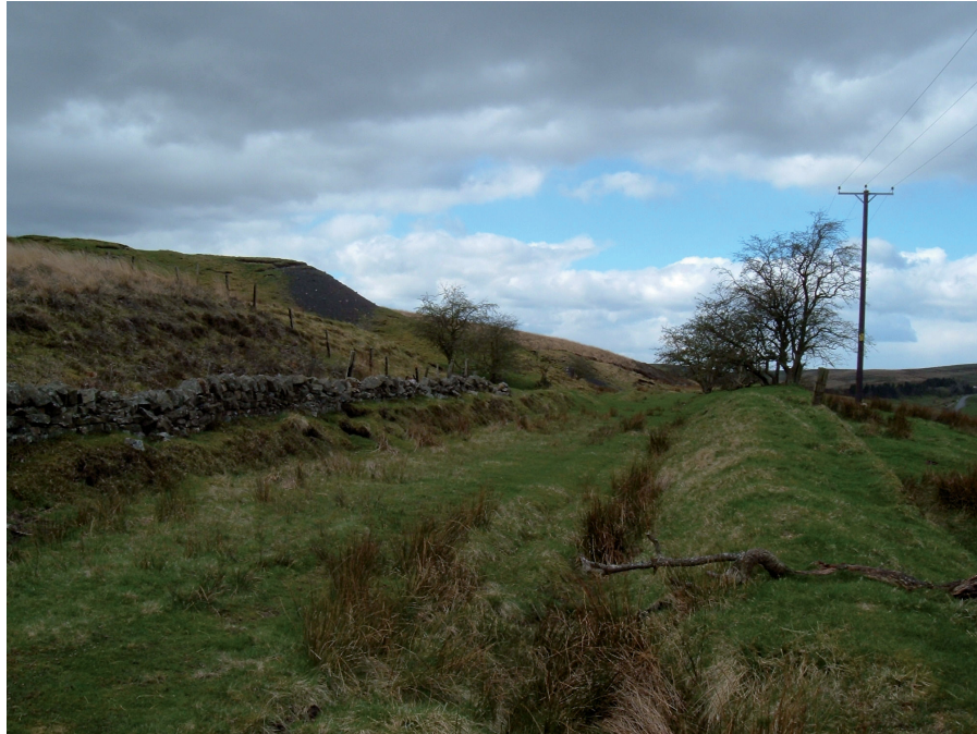
Plate 5: View from the east of trackbed and spoil heaps of Prior High Side Drift
