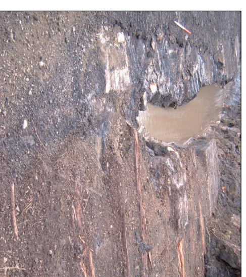
Remains of stone and concrete structures relating to the Tindale Granite Company on the south side of the trackbed
