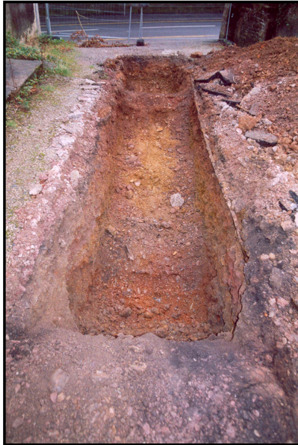
Plate 4: General view of Trench 2 from the north west
