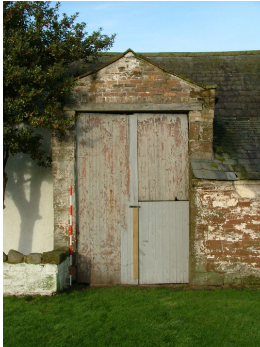
Plate 4 – Large doorway in south-east facing elevation of bank barn
