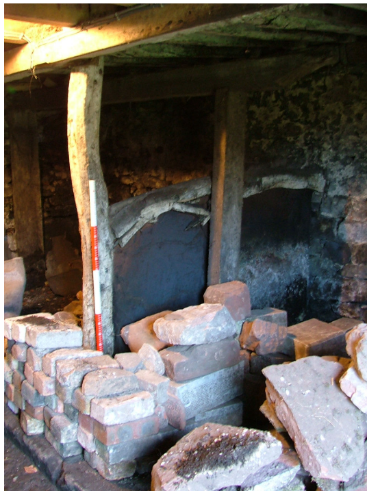
Plate 14 – Timber and sandstone stall division in byre
