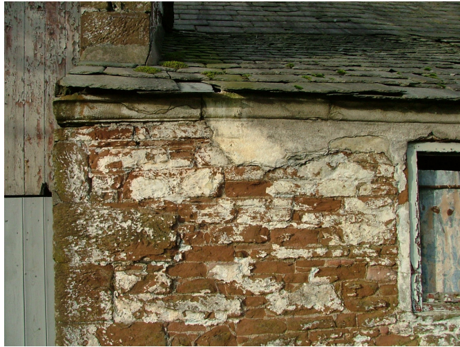
Plate 6 – Cornice of outshut (below slates), SE facing elevation of bank barn
