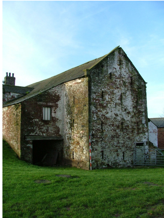
Plate 3 – North-east elevation of the bank barn, showing the coping stones and kneelers on the gable
