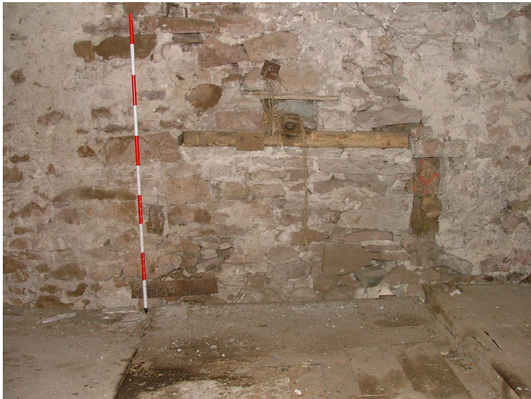
Plate 11 – Timber and niche in wall directly above the trapdoor
