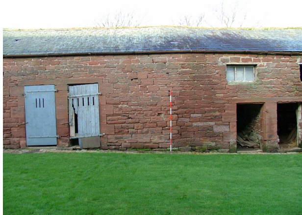
Plate 17 – Mid-section of stable block, facing courtyard
