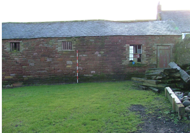
Plate 19 – Southern end of NW facing elevation of stable block
