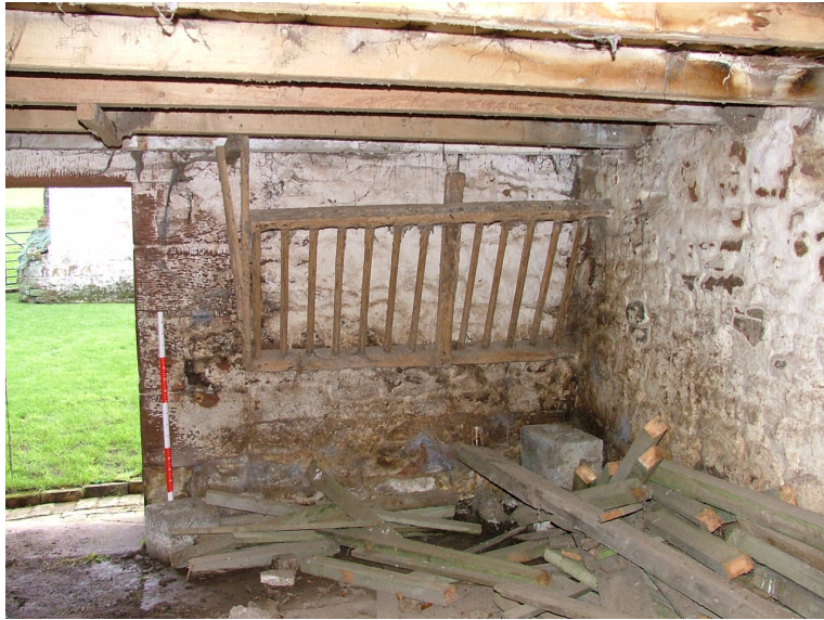
Plate 22 – Room (3) in stable block, showing the low ceiling and hay rack
