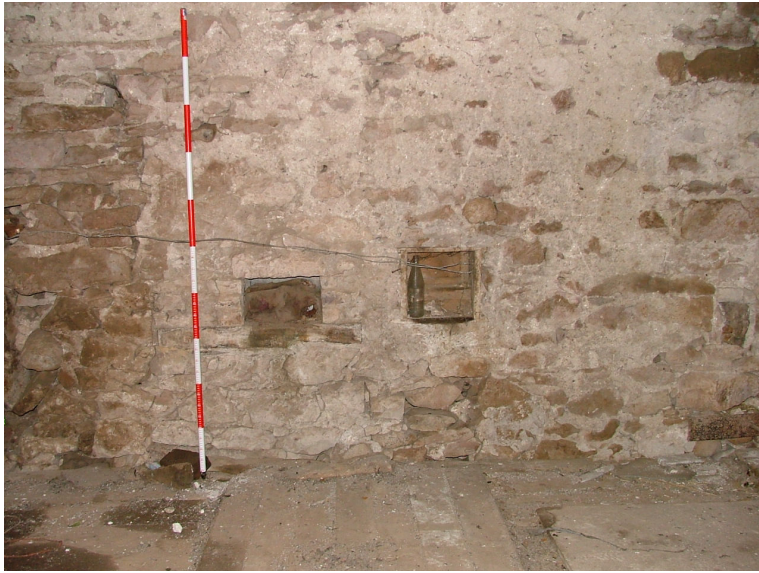
Plate 10 – Niches in the NW elevation of the bank barn
