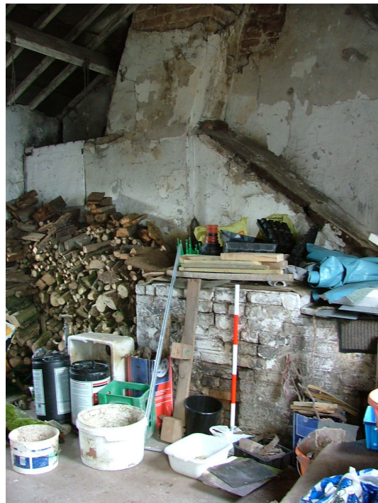
Plate 23 – Chimney breast in Room (6), stable block
