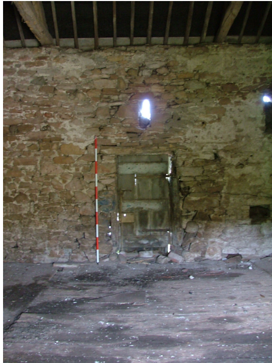
Plate 9 – Interior of bank barn, upper level, showing winnowing door and large timbers for the threshing floor
