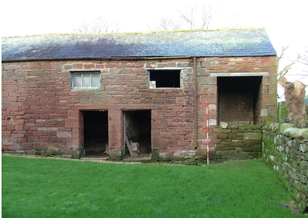
Plate 16 – NE end of stable block, facing into courtyard
