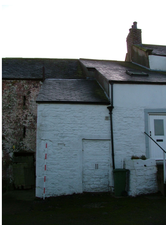
Plate 15 – Outshut of house with blocked-up doorway
