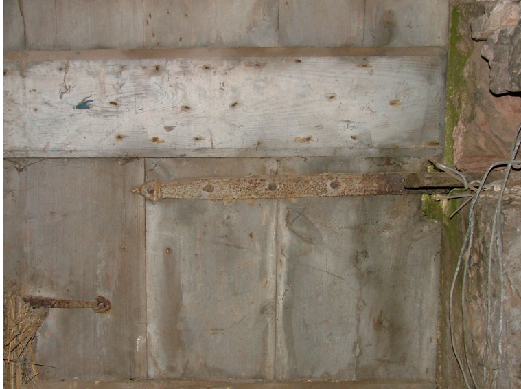
Plate 12 – Spearhead strap hinges, winnowing door of bank barn
