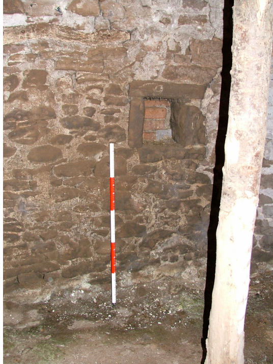
Plate 13 – One of the two blocked-up apertures, lower level of bank barn
