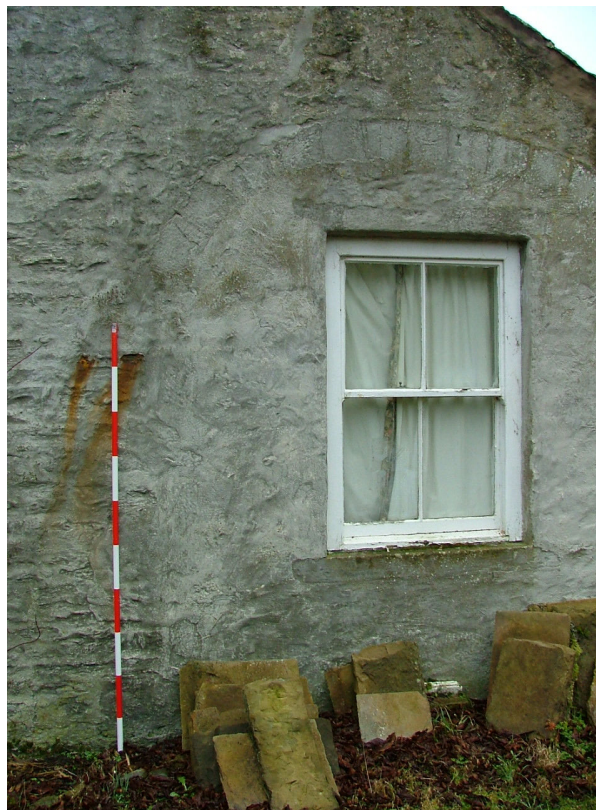
Plate 8 – Blocked-up archway, east elevation of farmhouse
