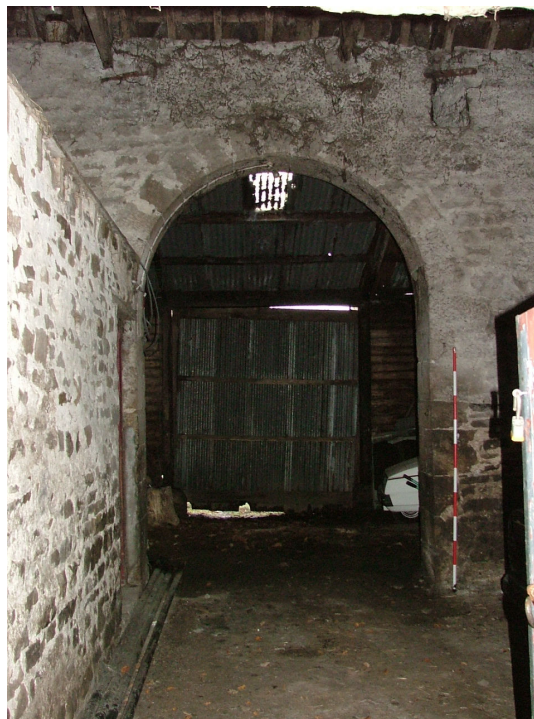
Plate 4 – Large doorway in northern elevation of barn
