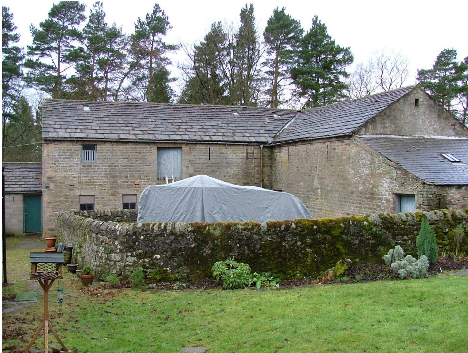
Plate 1 – The farm buildings as seen from the east
