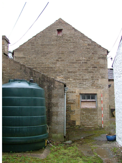
Plate 3 – South gable end showing blocked doorway
