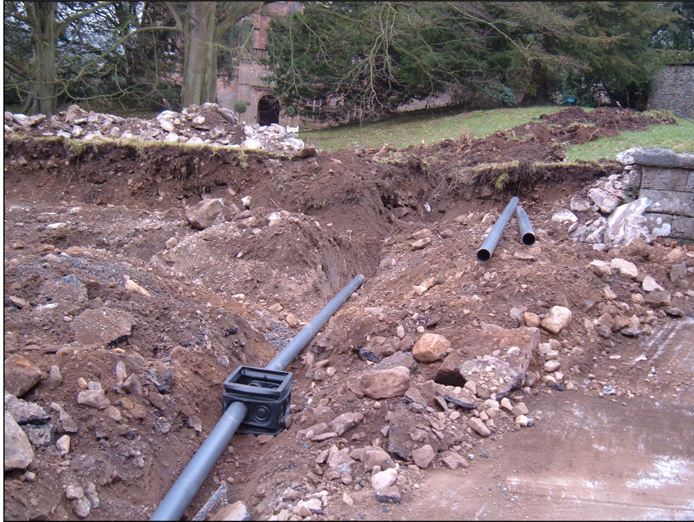
Plate 17: General Shot of drainage trenches, looking South-West. Photo: C.Jones
