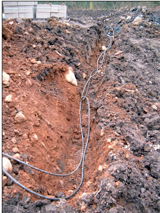
Plate 18: General Shot of drainage trenches, looking North. Photo: C.Jones
