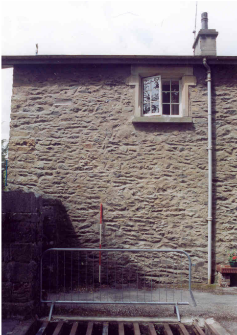
Plate 5: The Stable Block: South-East Elevation (southern end)
