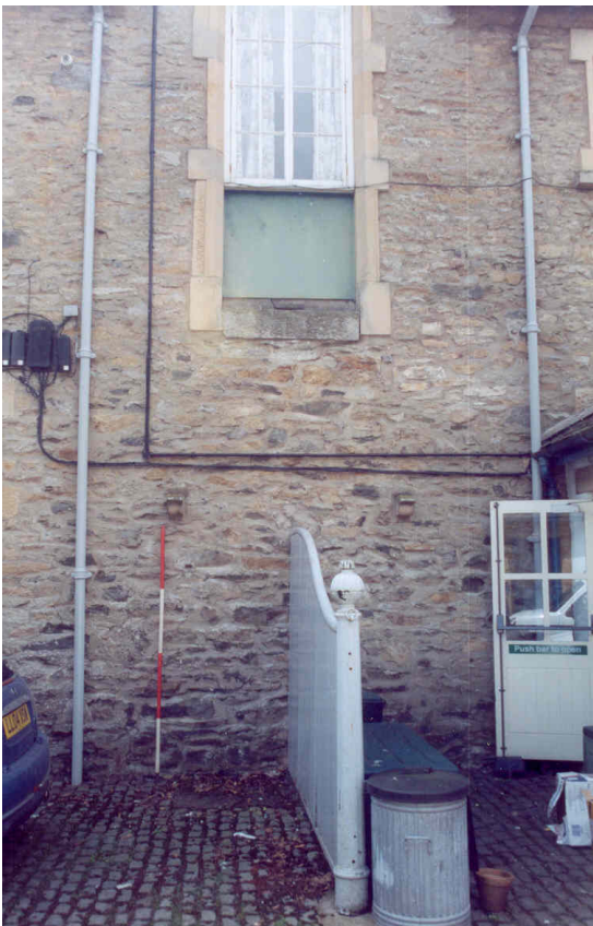
Plate 13: View of western bay of north facing elevation of central range, again illustrating later reduction in size of window
