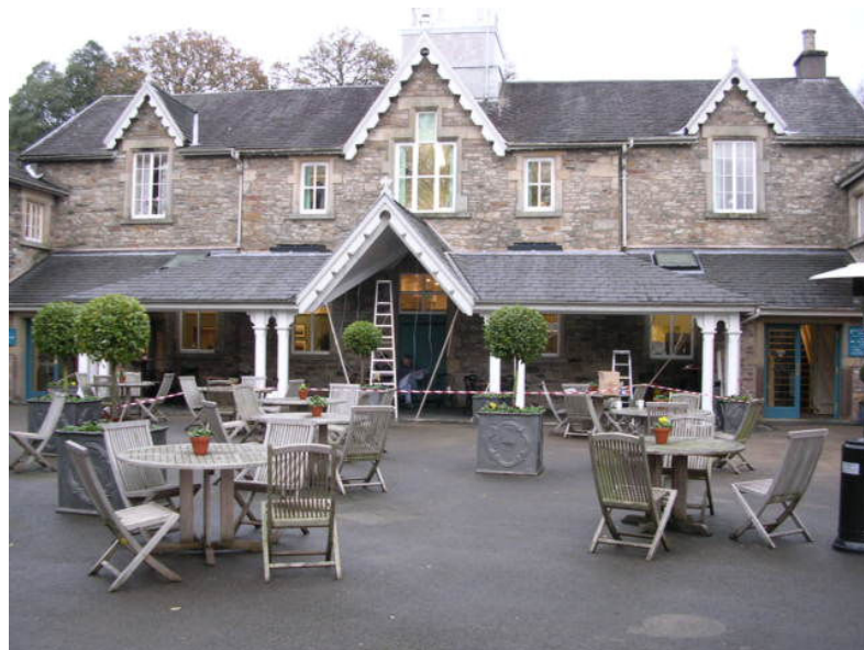
Plate 11: The Stable Block: General View of the South-West Elevation
