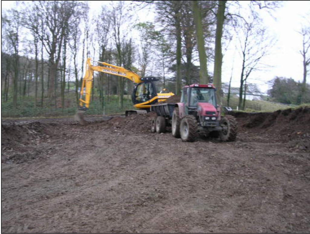
Plate 15: General shot of site stripping, looking North-East. Photo C.Jones
