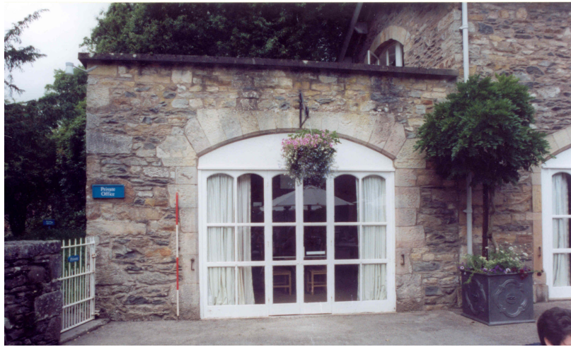
Plate 2: Later extension to the Stable Block: Internal Elevation looking North-West
