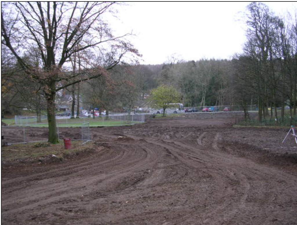
Plate 16: General shot of site stripping, looking west. Photo: C.Jones
