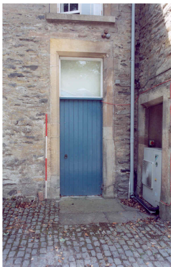
Plate 8: North west corner of main northern range.
