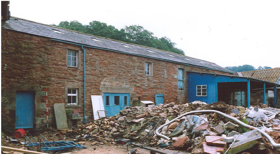
Plate 22 – Western elevation of Range C
