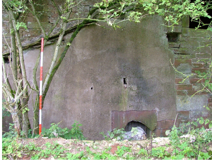
Plate 10 – West elevation, Range A – waterwheel axle hole and scarring of roofline
