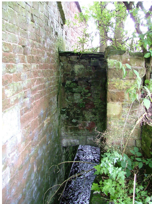
Plate 11 – Western elevation of Range A, mill race
