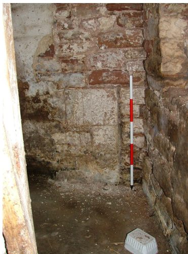
Plate 26 – Southern gable end of Range C, remains of quoins
