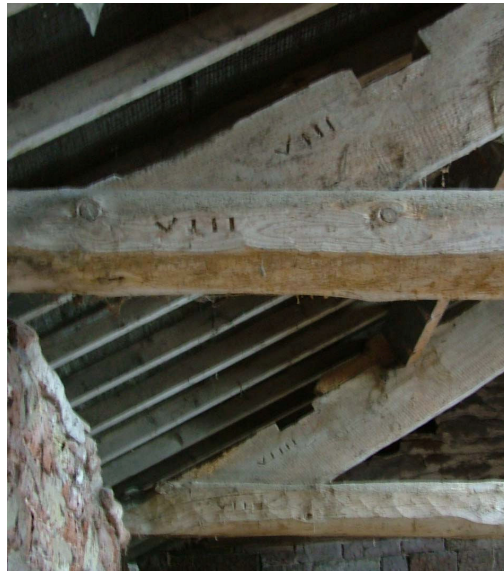
Plate 27 – Carpenter's marks – Range C
