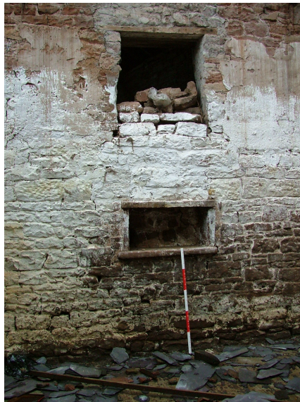
Plate 24 – Recess and window in gable – Range C
