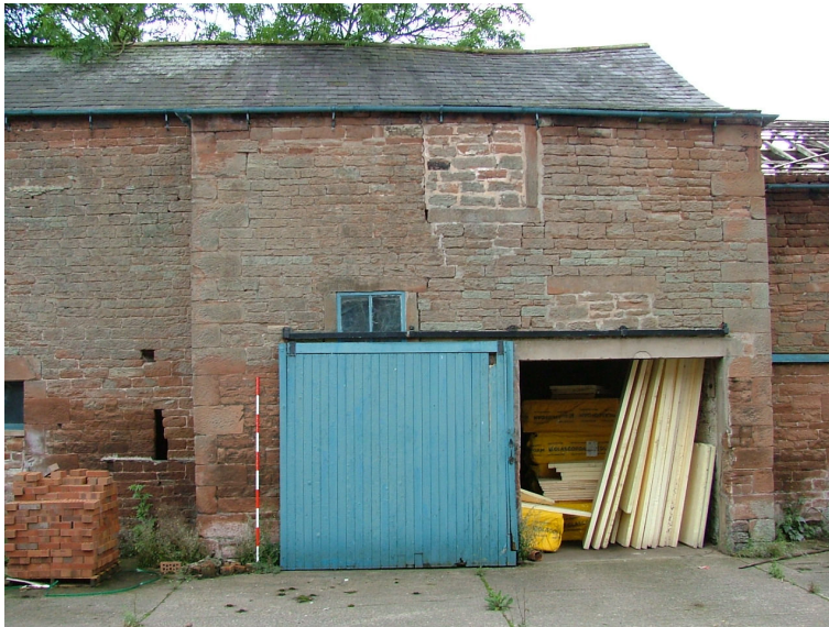
Plate 6 – Central section of Range A
