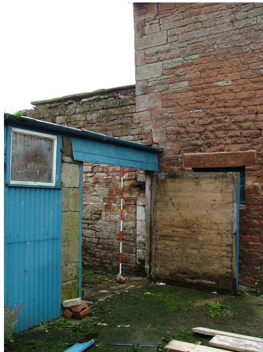
Plate 8 – Southern end of Range A, showing the wall built into the quoin
