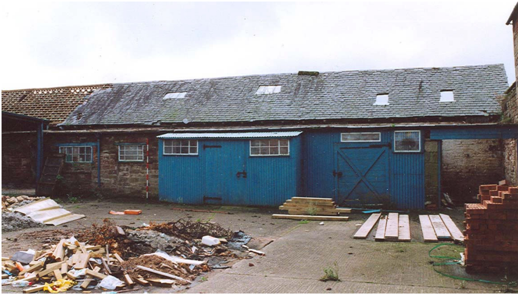
Plate 15 – Range B (Slated structure behind the later lean-to)
