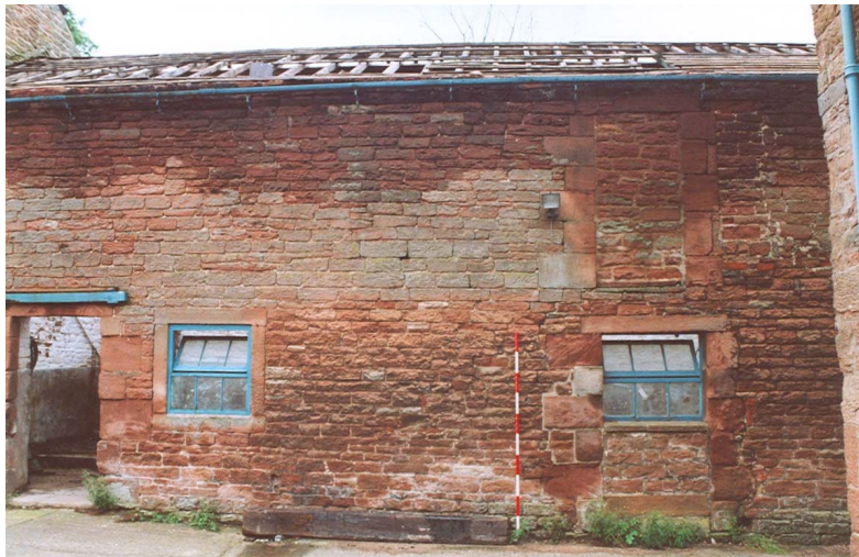
Plate 4 – Eastern elevation of Byre, Range A
