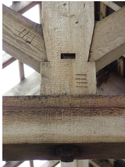
Plate 20 – Carpenter's (or assembly) marks on a roof truss in Range B
