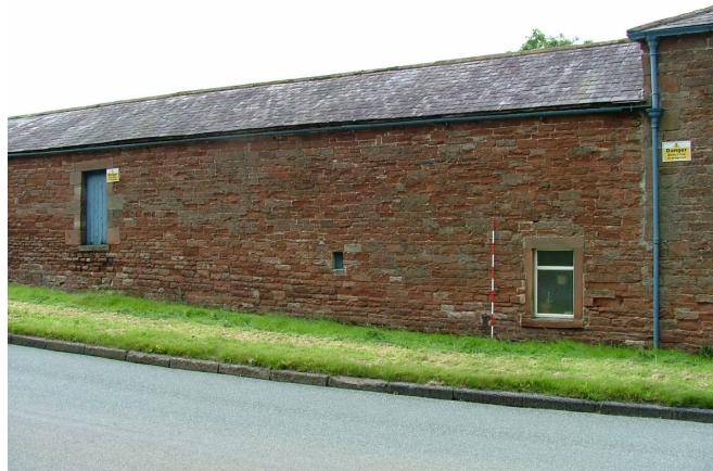
Plate 23 – Eastern elevation of Range C
