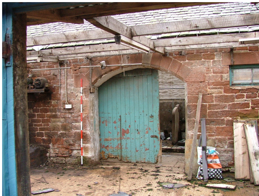
Plate 17 – Range B, arched doorway at eastern end of northern elevation
