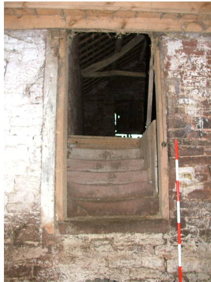
Plate 12 – Doorway in Range A, gives access to the bank barn
