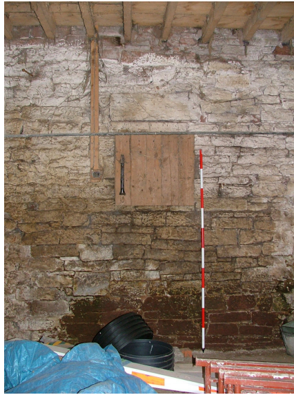
Plate 13 – Wooden door covering axle hole, Range A
