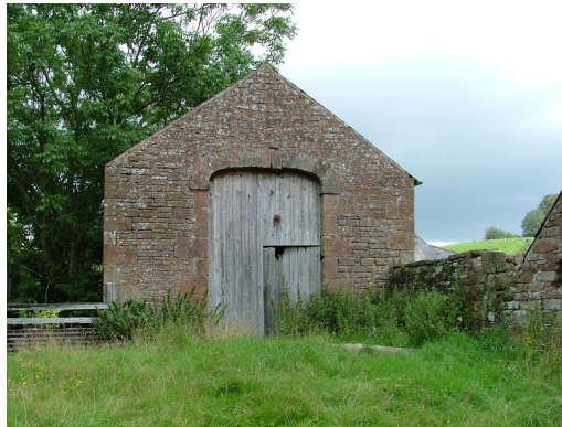
Plate 9 - Large doorway in southern gable end of Range A
