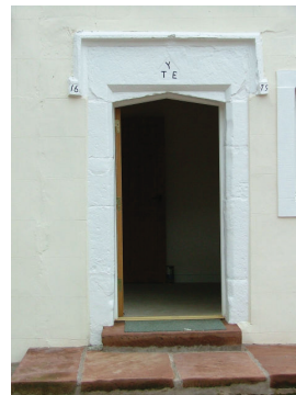
Plate 10 – Doorway – rear entrance
