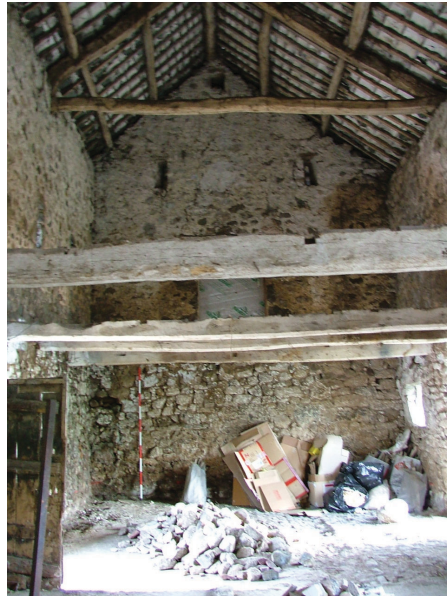
Plate 4 – Northern gable end of Building A
