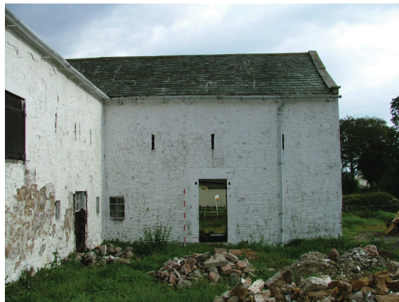
Plate 5 – Southern elevation of Building B
