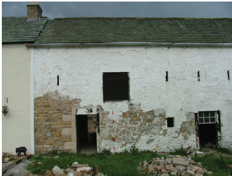
Plate 2 – Building A, Eastern Elevation
