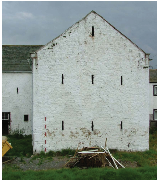
Plate 6 – Eastern gable end of Building B
