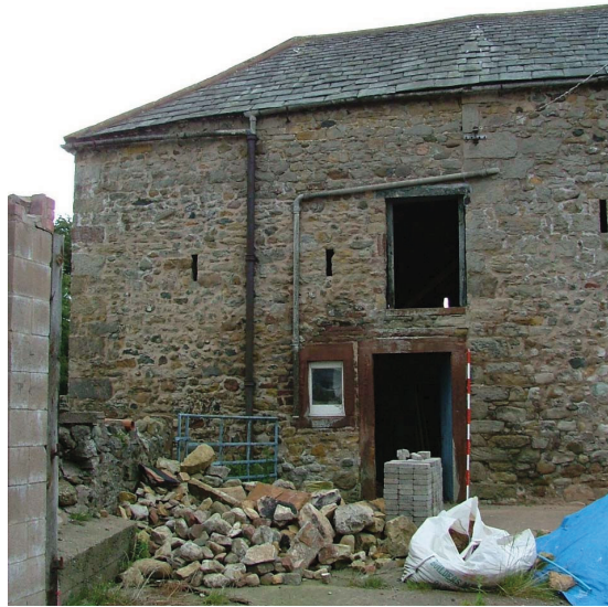
Plate 8 – Western gable end of Building B
