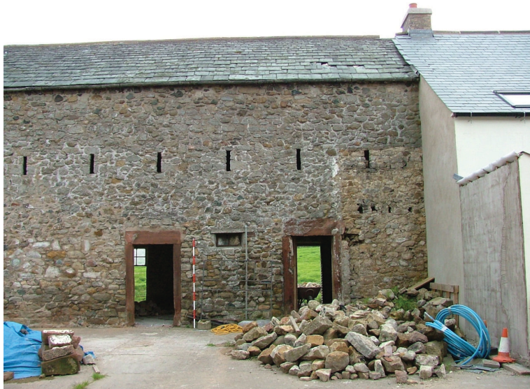
Plate 3 – Western Elevation of Building A
