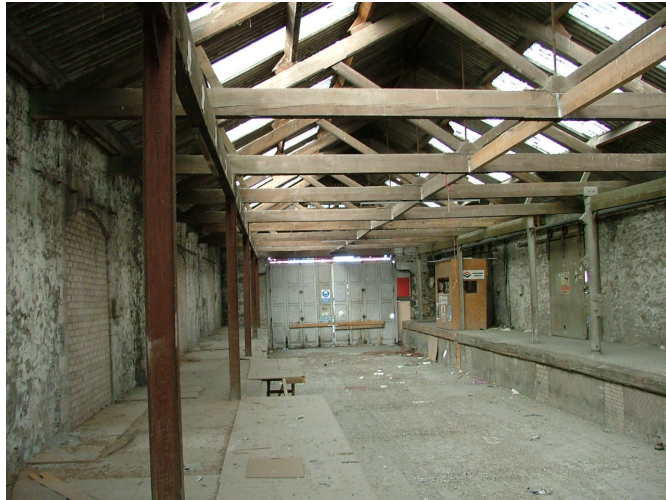
Plate 19 – Roof structure of central range – note the central timber 'binders' joining all the tie beams below the base of the iron rods, and the vertical girders on the left and pillars on the right-hand side platform
