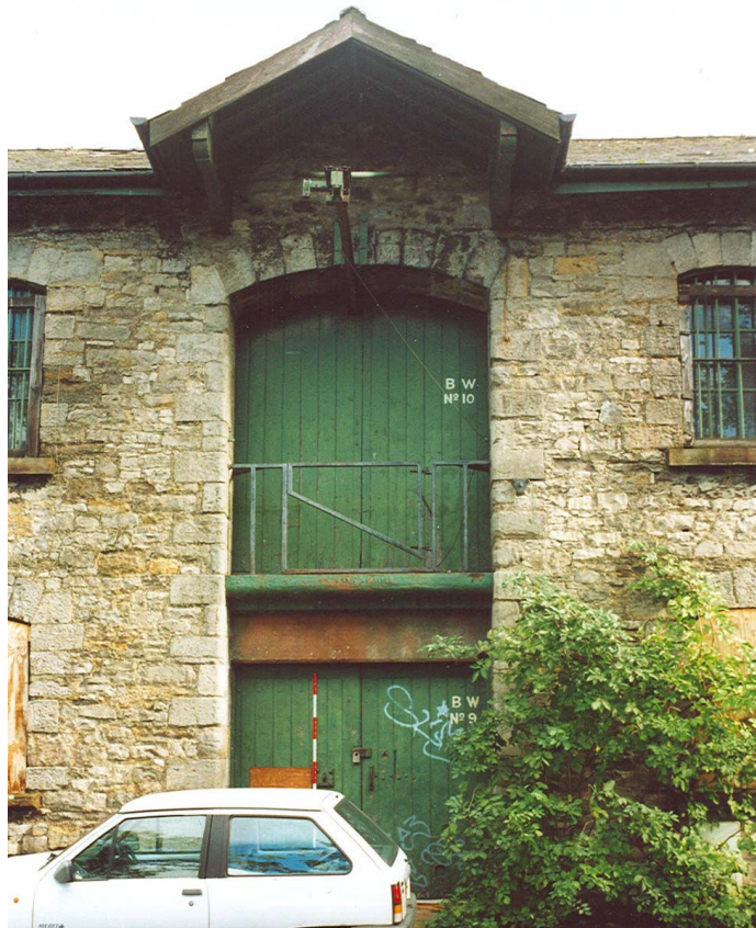
Plate 5 – SW Elevation, View of doorways with sandstone and cast iron lintels and hoist still in-situ
