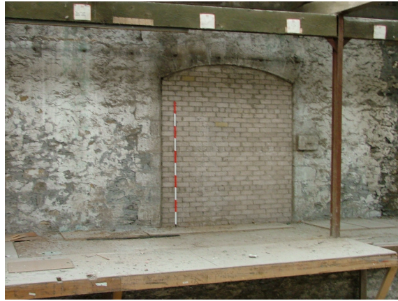
Plate 17 – Blocked-up doorway of western range, as seen from the central section
