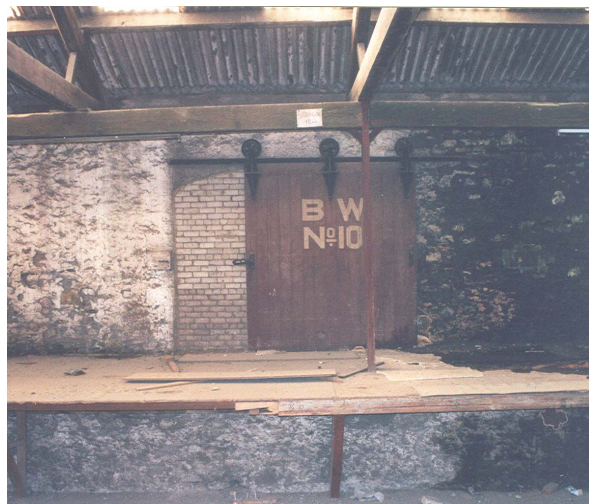
Plate 18 – BW No.10 door (western range) still in-situ , although blocked-up behind, as seen from the central section
