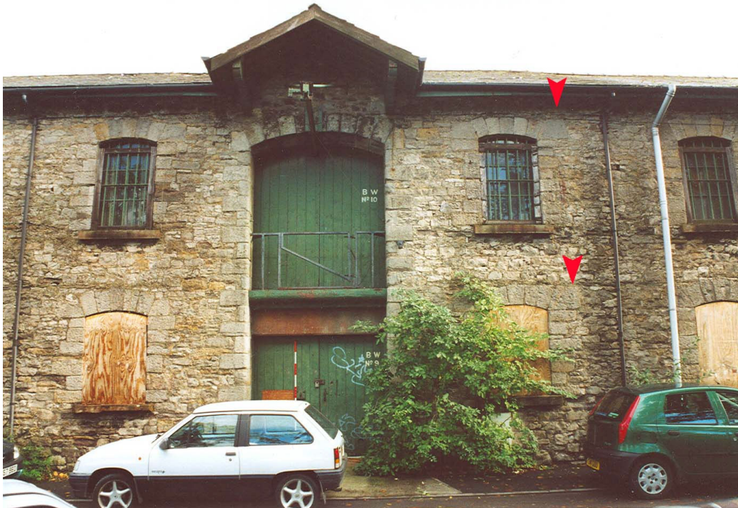
Plate 3 – SW facing elevation – Red arrows indicate the layers of slate
