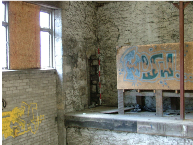
Plate 21 – The western (blocked) of the two doorways in the SE elevation, originally accessed via external stairs into the central section of the warehouse
