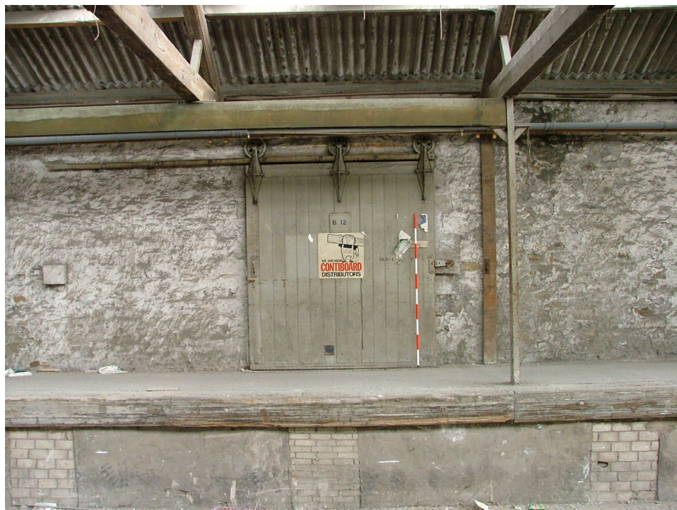
Plate 14 – View of large sliding door in wall between the central and western ranges, showing the sliding mechanism and the large stone to the left, which prevents the door from sliding off its rail
