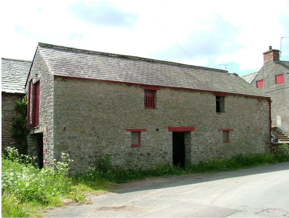
Plate 10 – NW Elevation of Building 3
