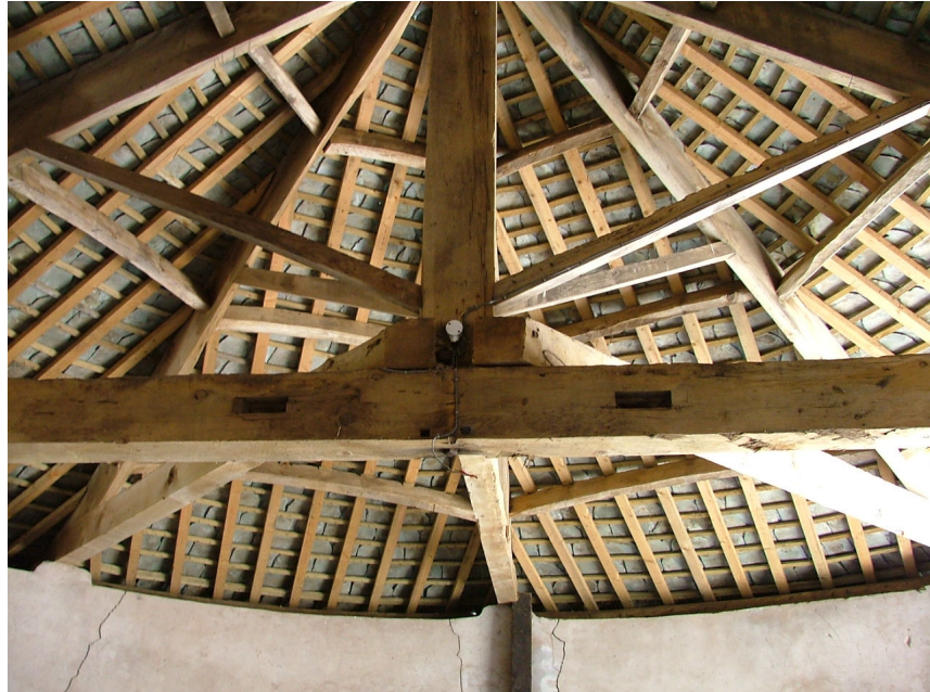
Plate 8 – Roof structure of gin-gang
