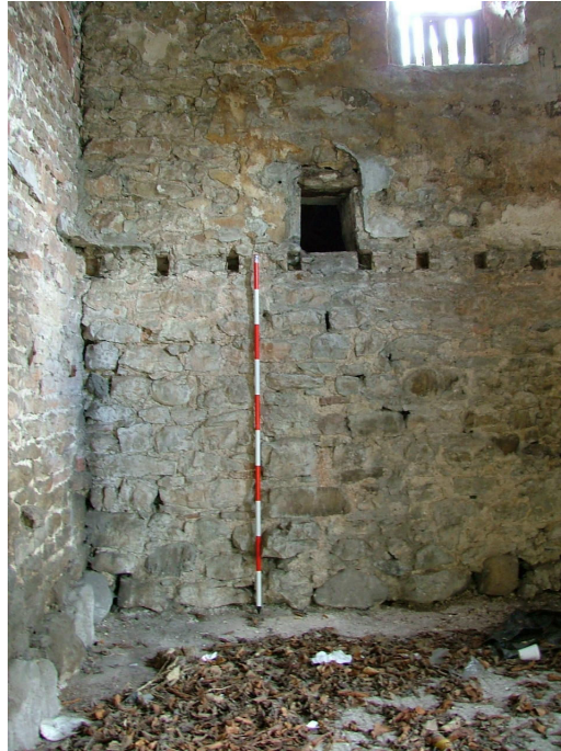
Plate 12 – Joist holes and ‘vent’ in Building 3 (SW end)
