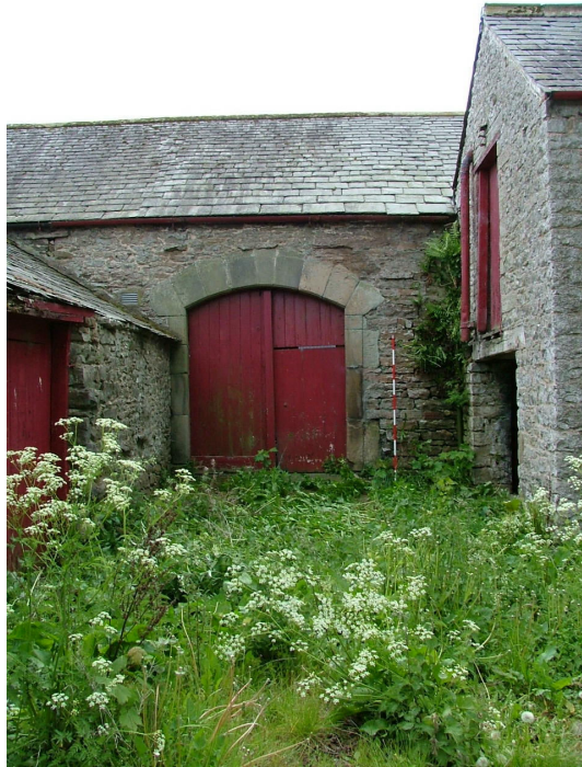
Plate 4 – Doorway on north-western elevation
