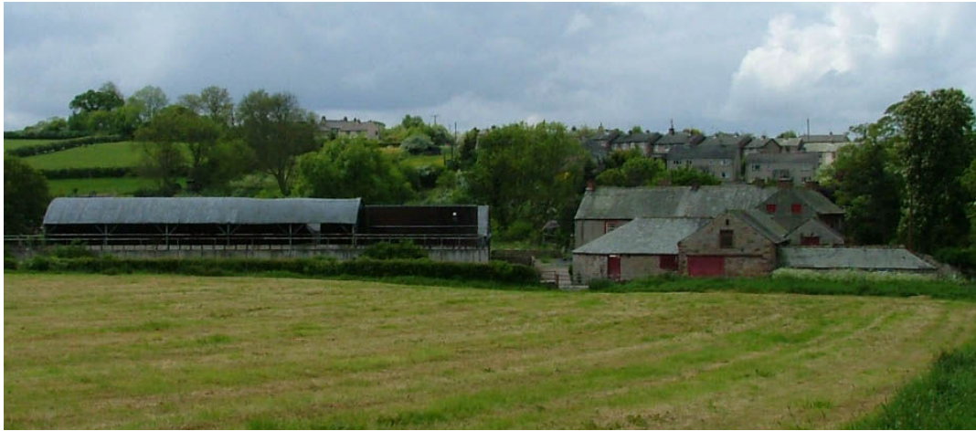
Plate 1 – Hall Farm, Morland from the north-east. The range of farm buildings is visible on the left of the photograph.
