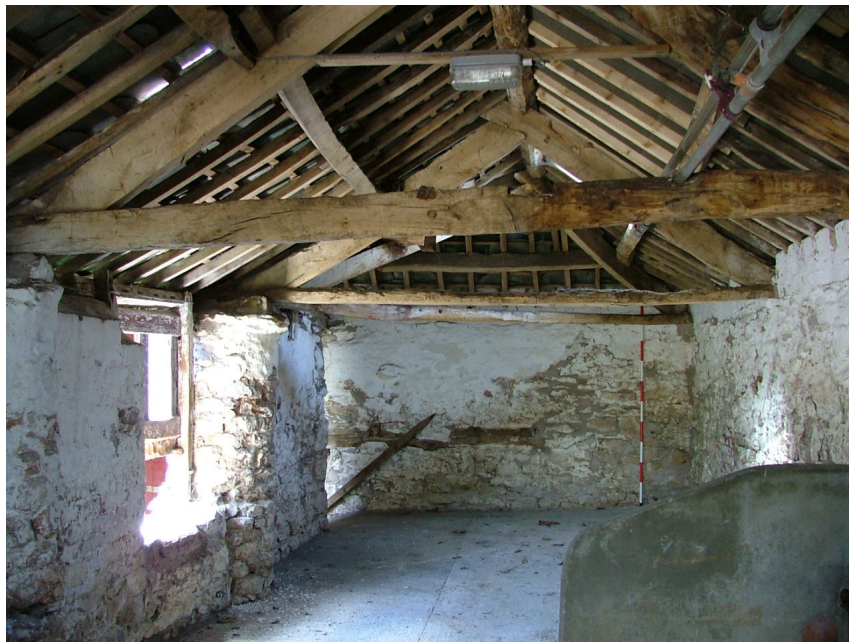
Plate 14 – One of the ranges in Building 4, on the left are the circular stone piers that support the roof.
