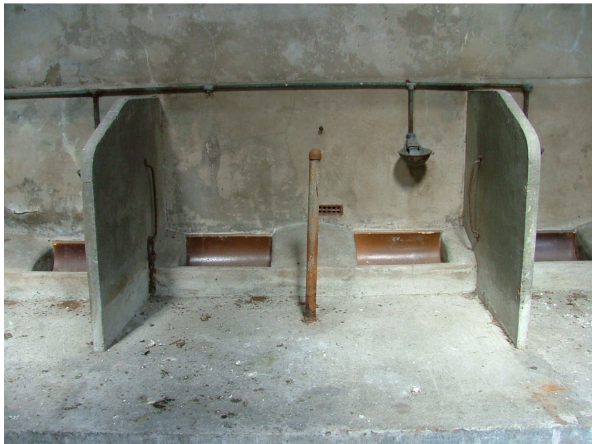
Plate 5 – Concrete double stall in Building 1
