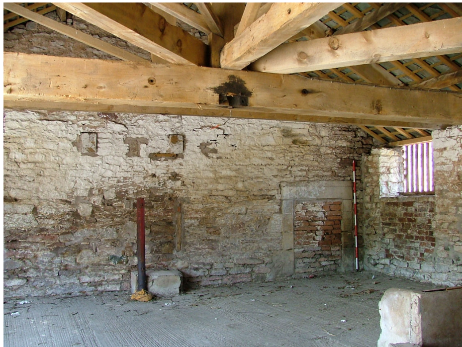
Plate 7 – Interior of gin-gang showing blocked doorway and ventilation slits
