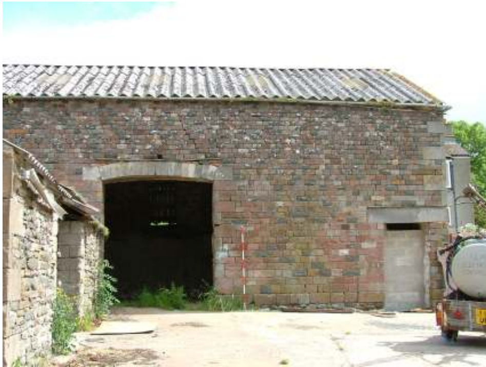
Plate 2: South-west facing elevation of Barn A
