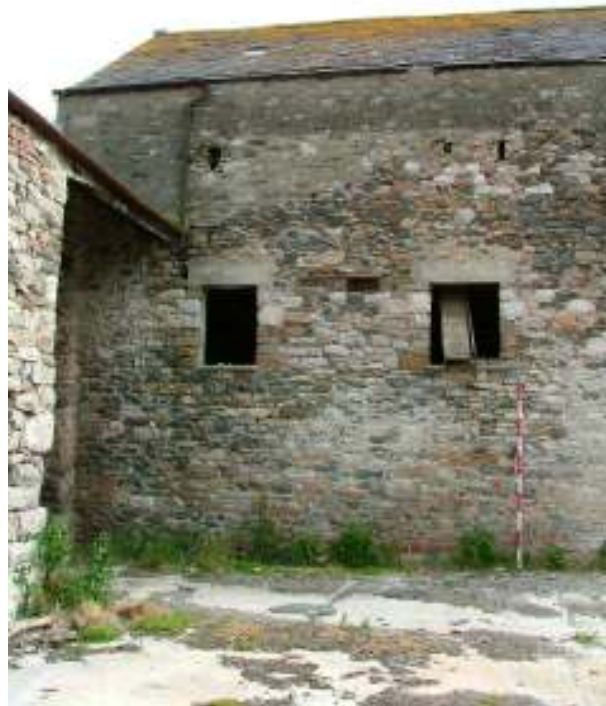
Plate 16: South West facing elevation of Building 4, shows wooden chute and scarring of a demolished building
