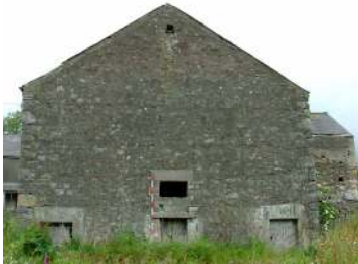
Plate 11: South West facing gable end of Barn B – showing 3 doorways
