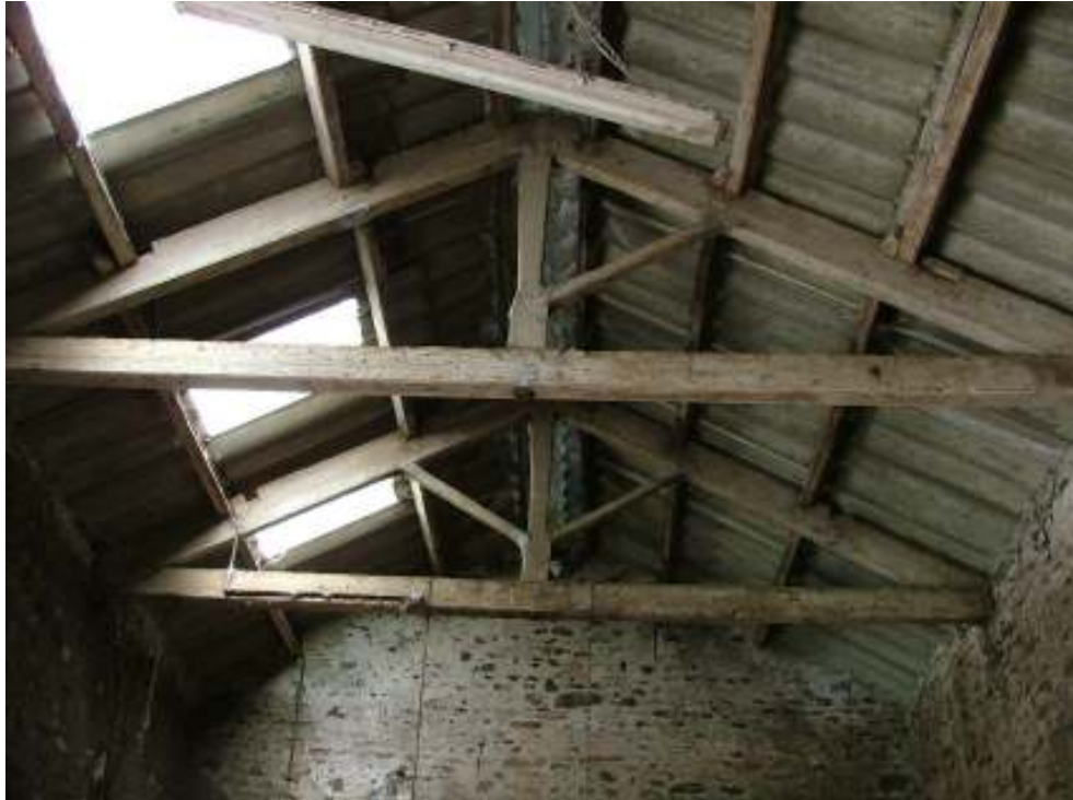
Plate 4: Roof structure in Barn A
