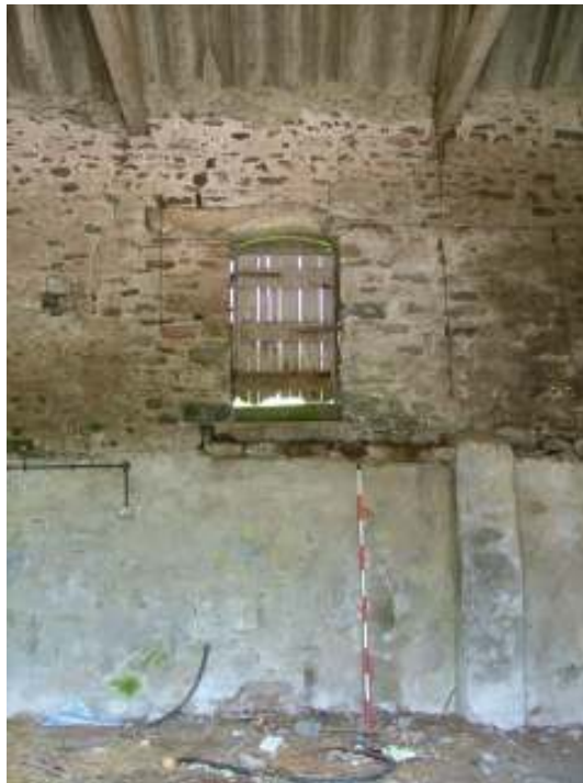
Plate 5: Barn A, first floor doorway
