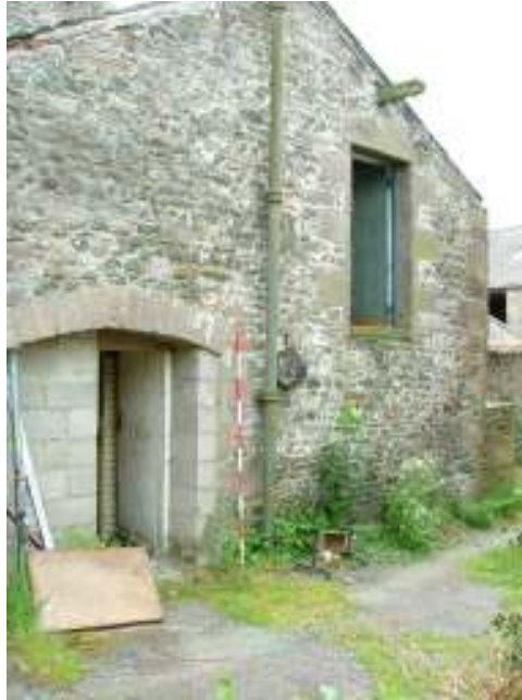
Plate 6: North West facing elevation of Building 1
