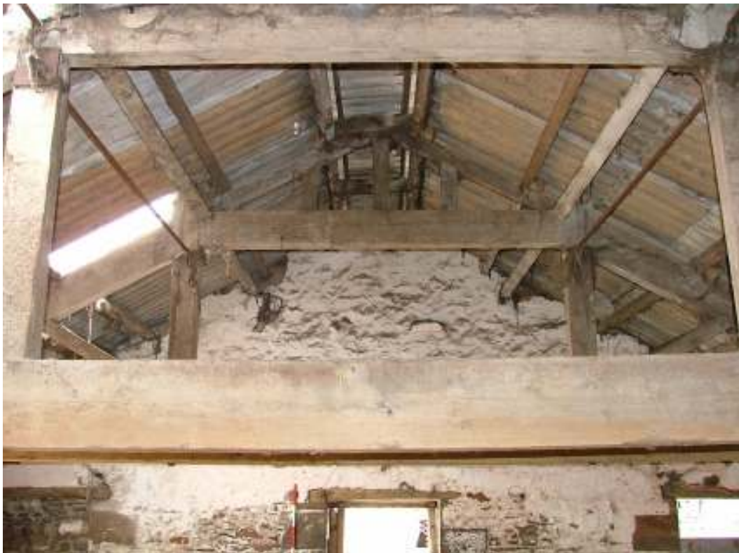
Plate 9: Queen-post roof structure in Building 2
