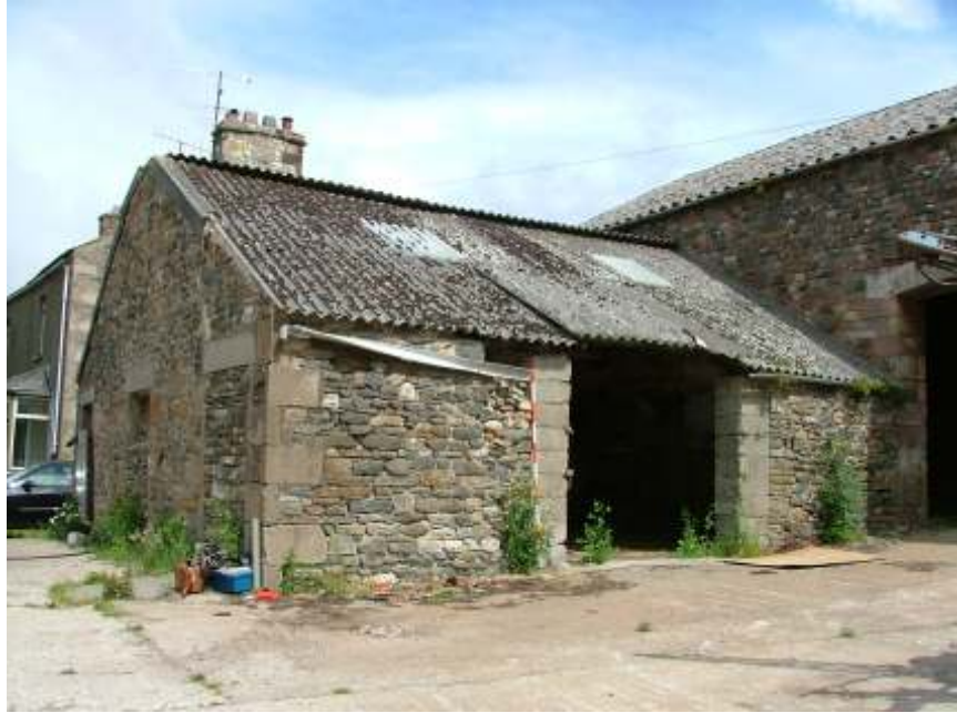
Plate 7: Building 2 from the south
