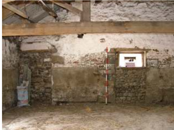
Plate 8 – Interior of Building 2 showing blocked doorways
