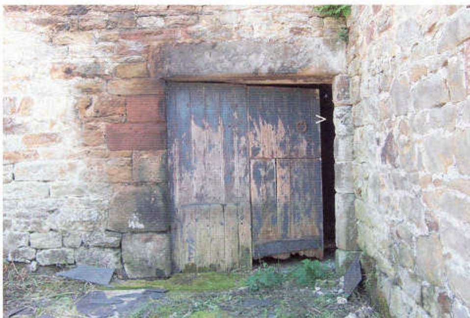
Figure 10 The main entrance to the Phase 1 building. The arrow points to the stone of the right-hand door jamb with the inscriptions hidden behind the Phase 2 extension wall. (photograph: F. Wooler)
