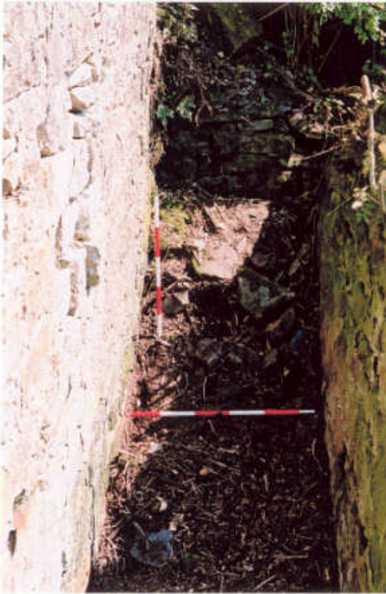
Figure 13 The wheel pit viewed from the north-west. It has been cleared of vegetation and debris but not bottomed. The scales measure one metre. (photograph: P. Cracknell)
