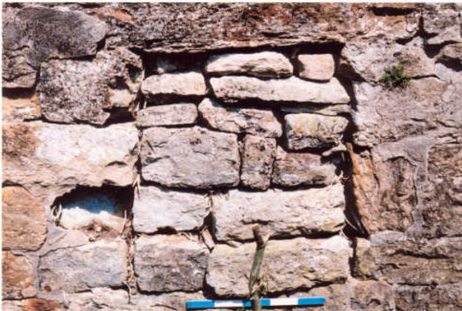
Figure 14 The blocked opening for the drive shaft of the water wheel in the south-western gable of the Phase 1 building. The scale measures 500 millimetres. (photograph: P. Cracknell)
