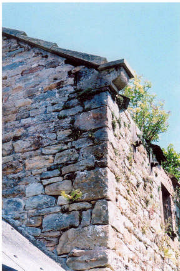
Figure 9 The kneeler and stepped gable coping on the Phase 2 extension. (photograph: P. Cracknell)
