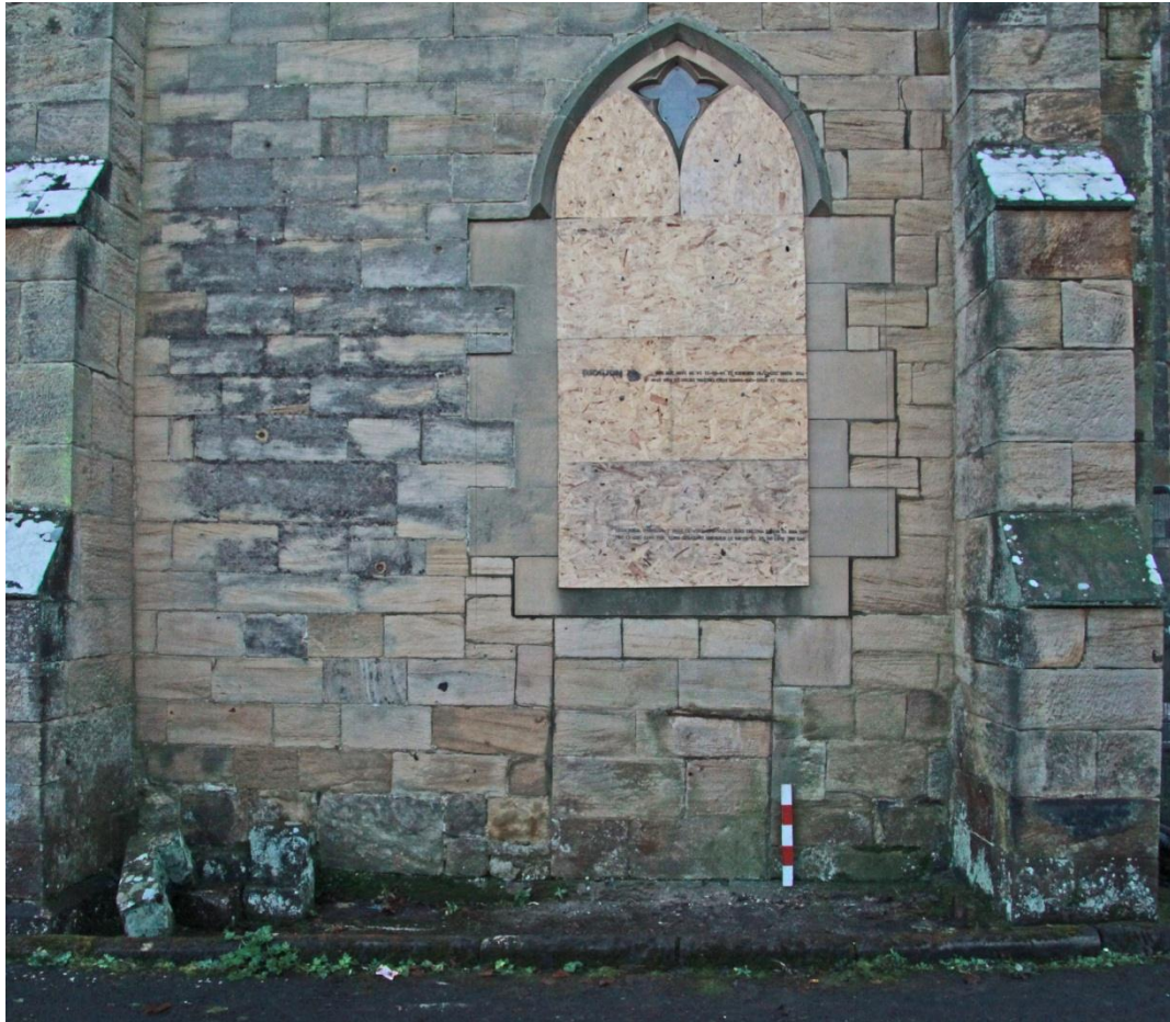
The exterior of the north wall, before works
