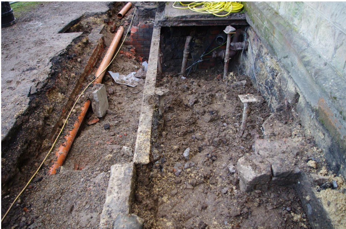
Illus vii. Remains of Boiler Room looking east
