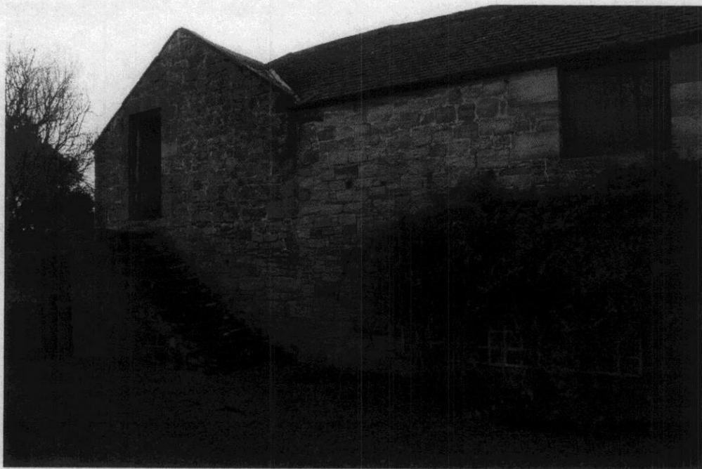
Range A (and north end Range B) from north-west
