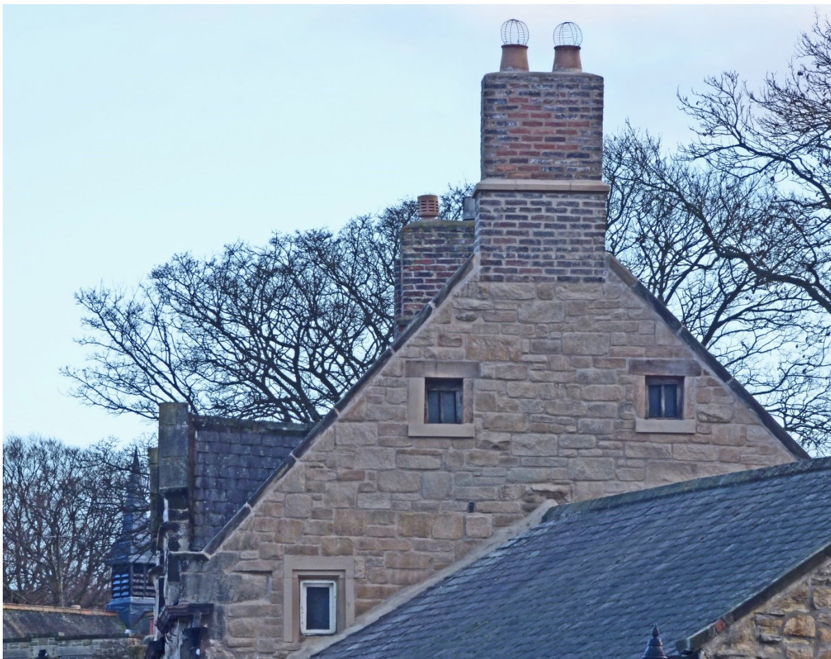
(14) North gable end after works, February 2016
