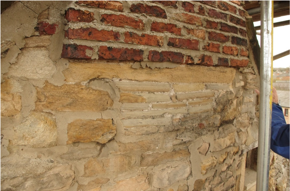
(7) Base of stack before works
