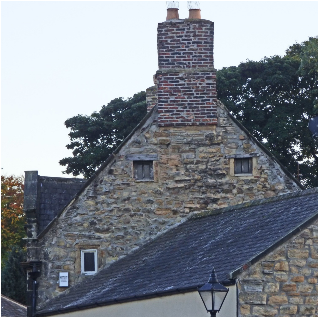
(2) North gable end before works, November 2015 (P2)
