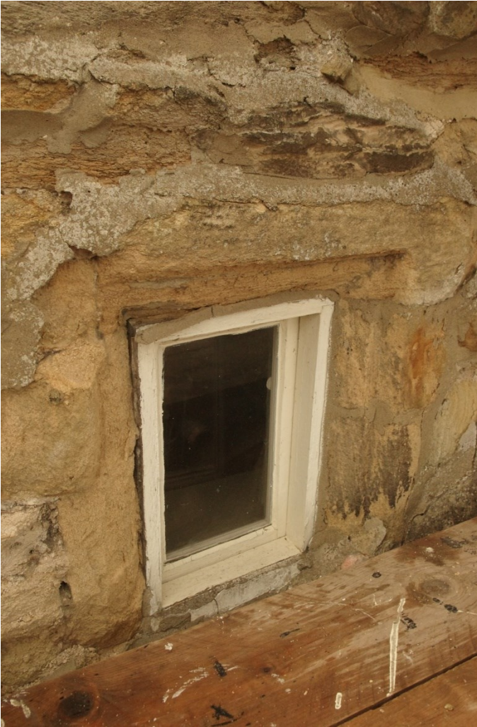
(4) Attic window in north gable end before works.
