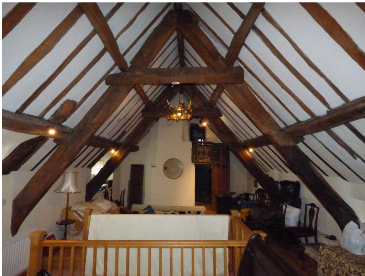
(16) Second (Attic) floor looking north showing upper cruck roof trusses (P16)
