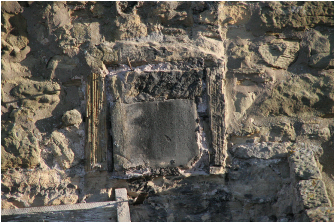
The newly-exposed window in the west gable
