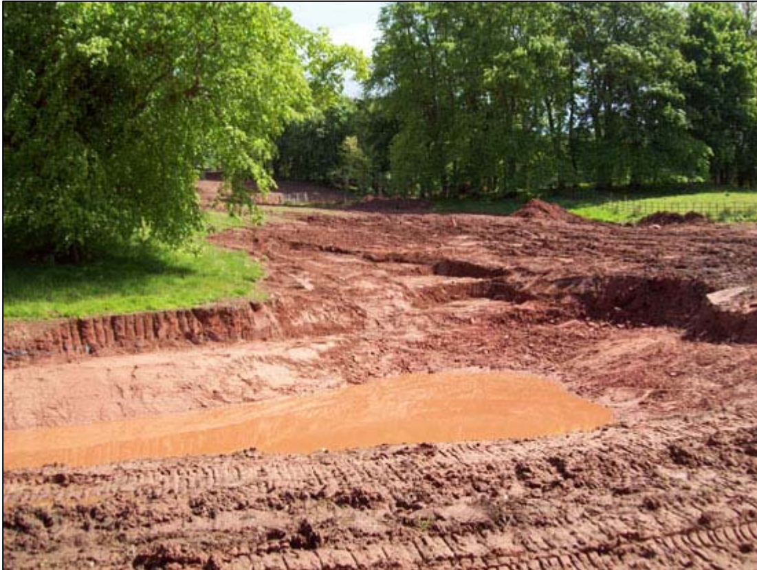
Figure 4a: Excavation for the Pond
