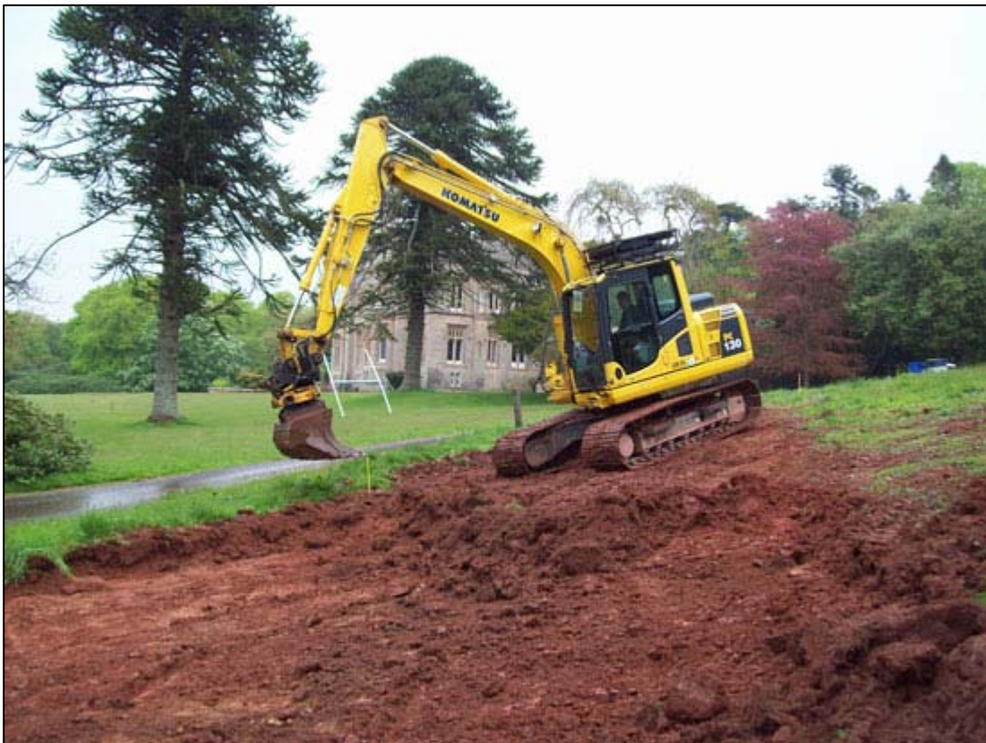
Figure 4b: Excavating for the Ha-ha
