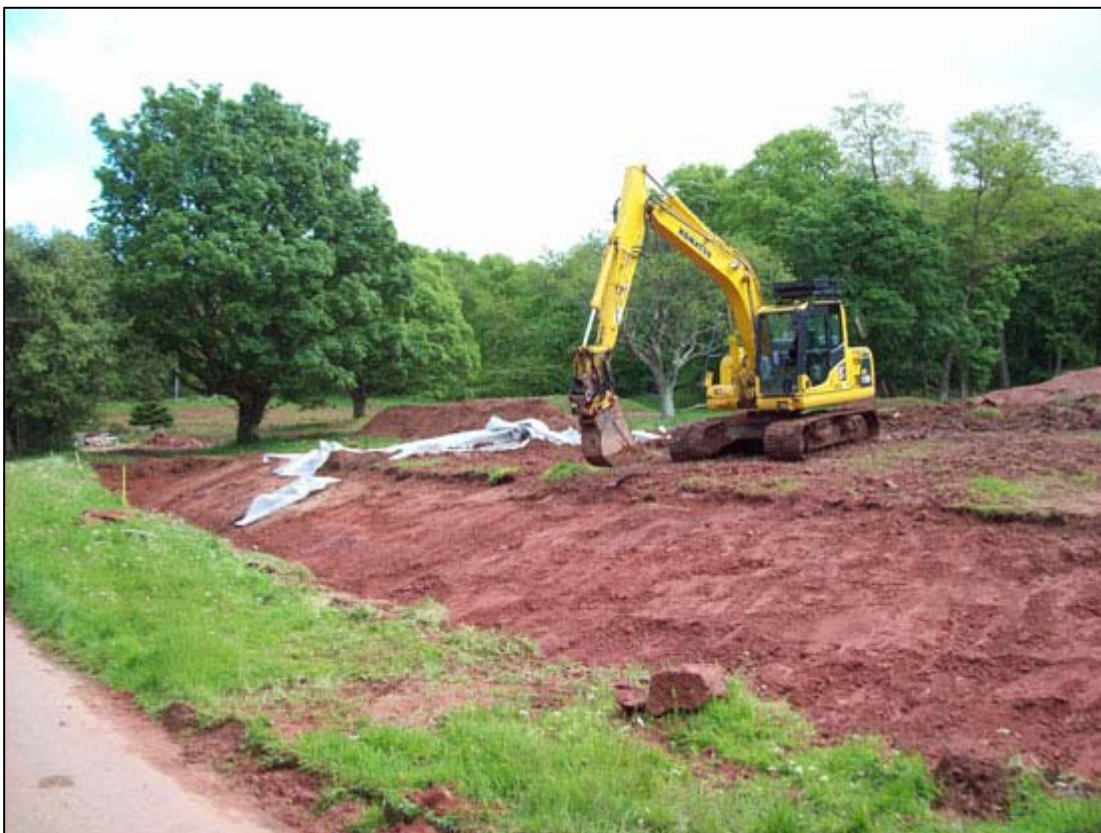
Figure 5b: Excavating for the Drainage
