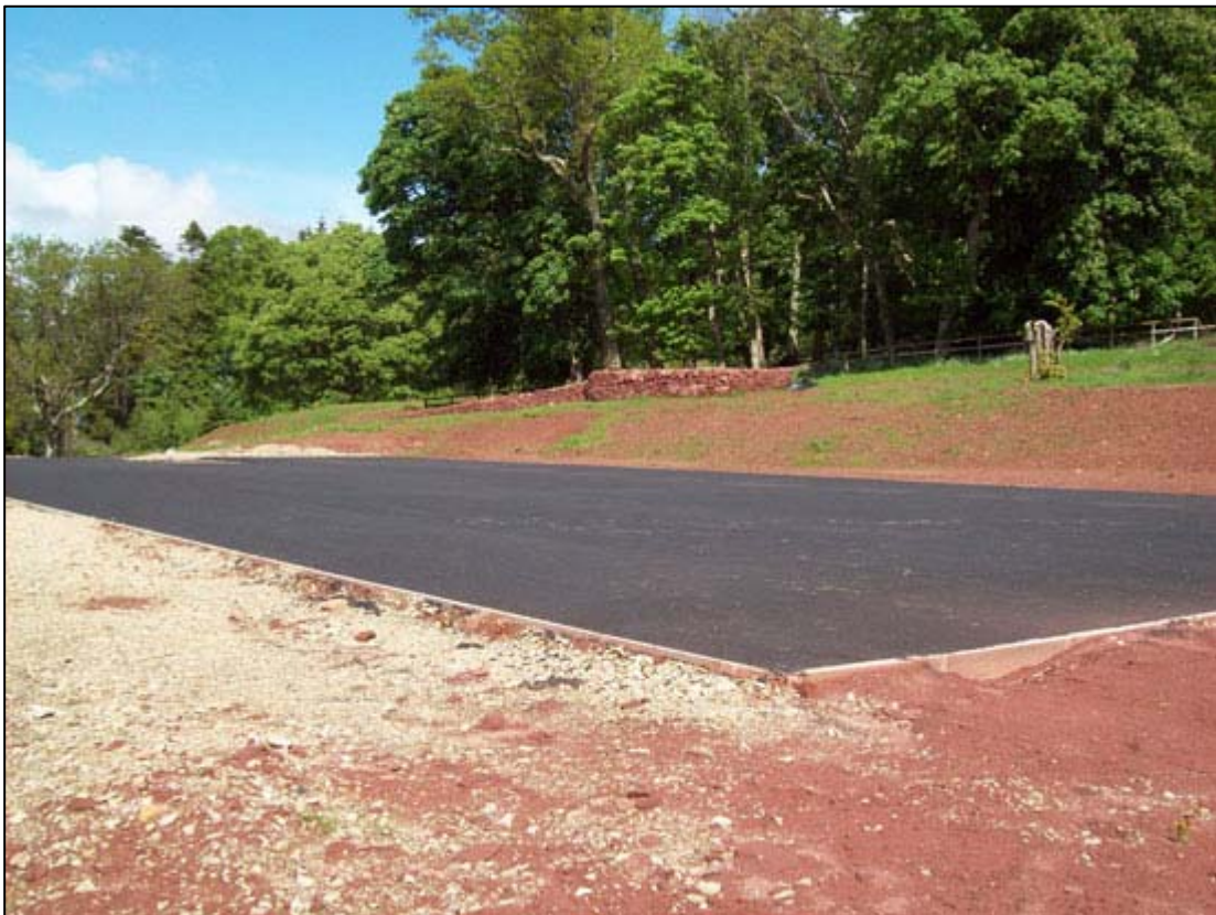
Figure 3b: Excavation for the Tennis Court and Pavilion
