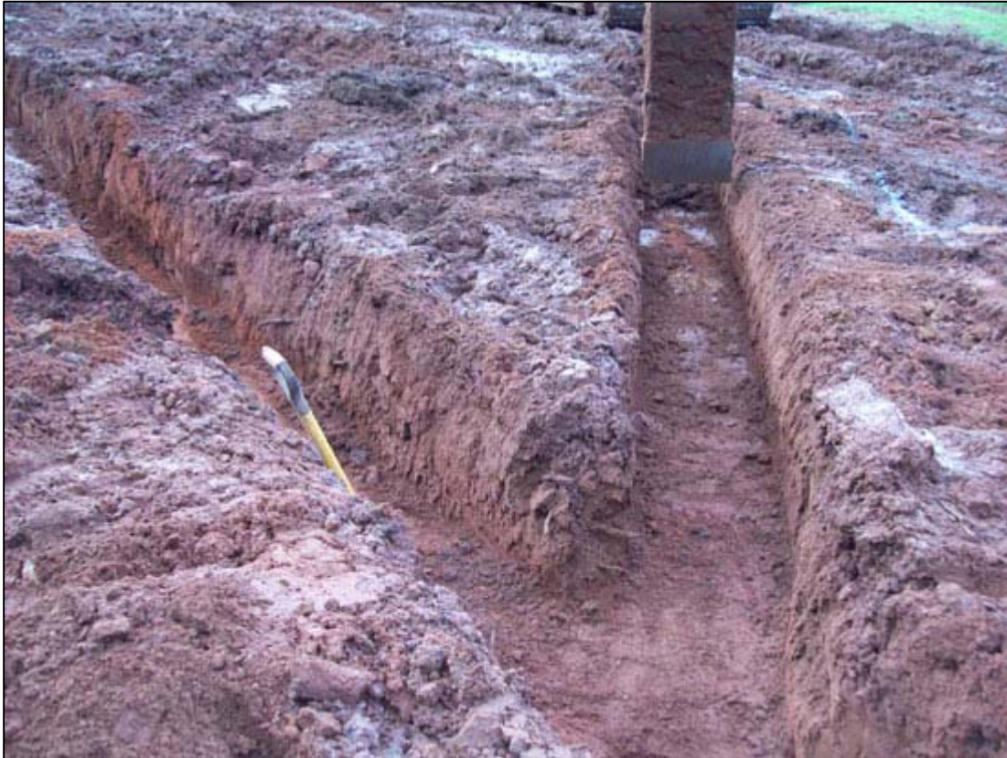
Figure 6a: Drainage tracks
