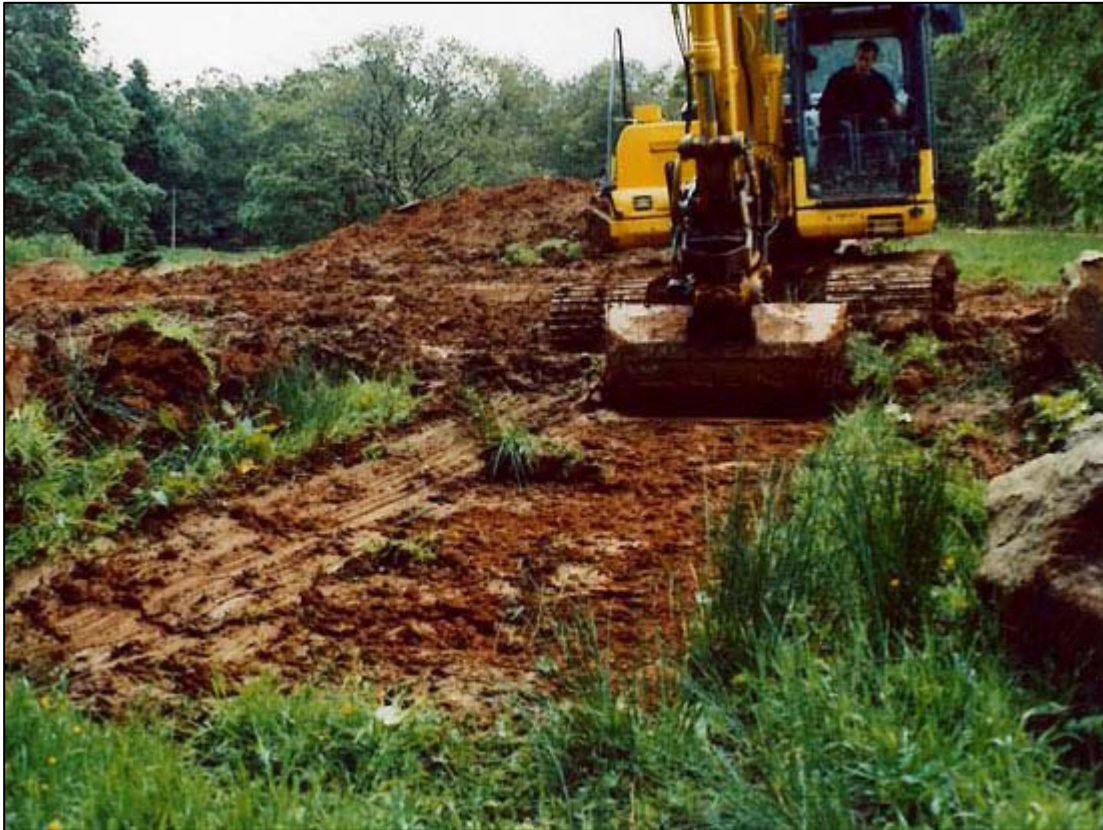
Figure 7a: Area stripped for access
