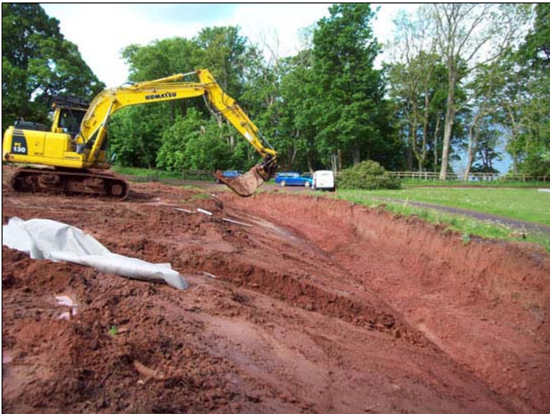
Figure 6b: Excavating Drainage near Ha-ha
