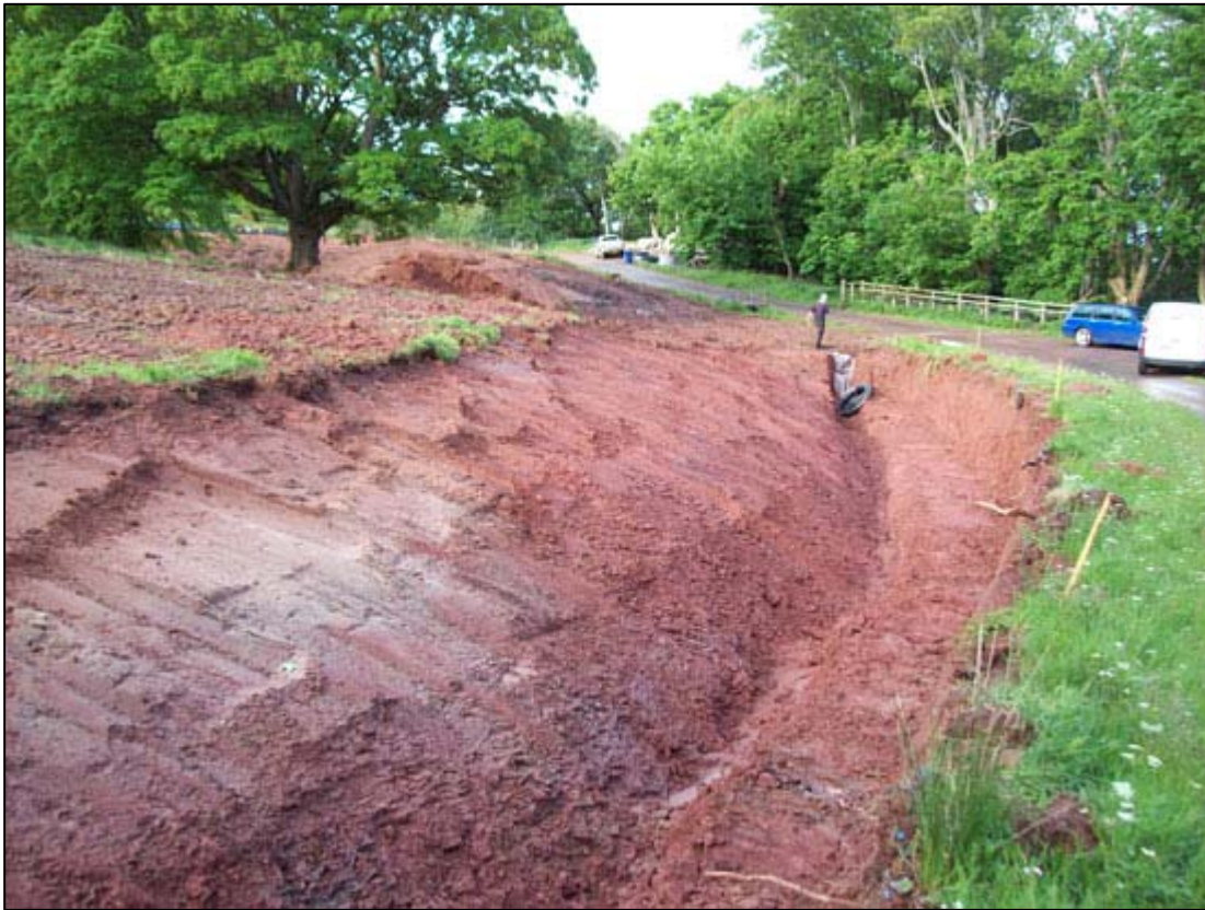
Figure 5a: Completed excavation for the Ha-ha
