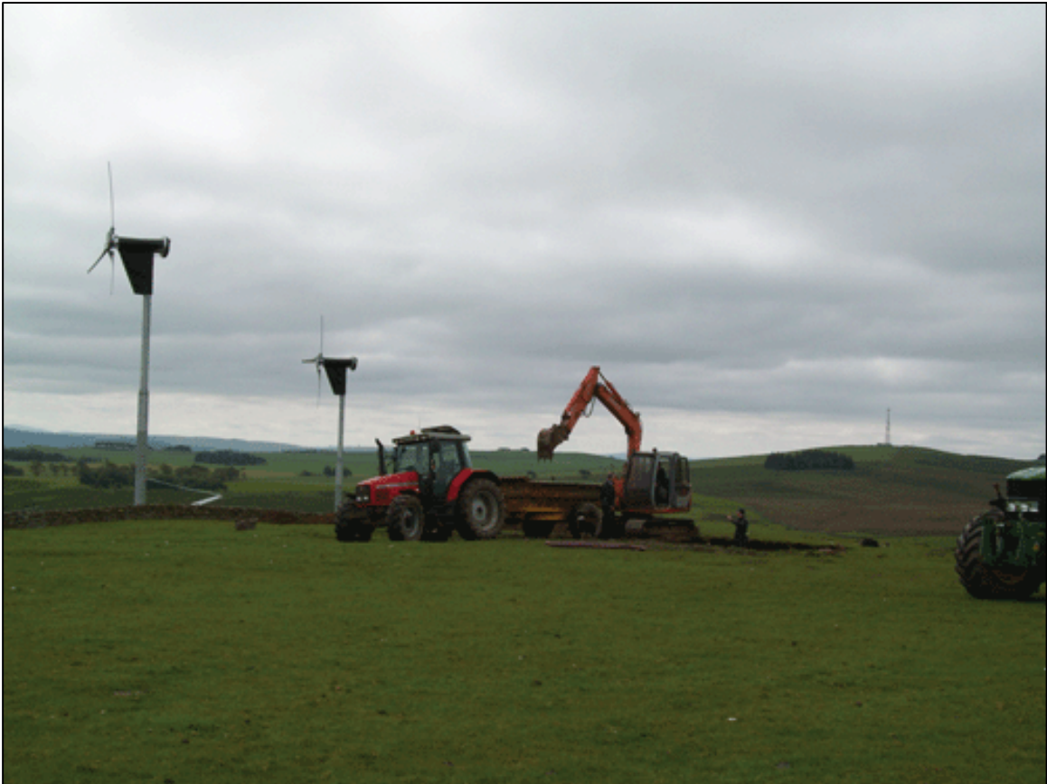
Figure 3a: General shot of site from the north-north-east
