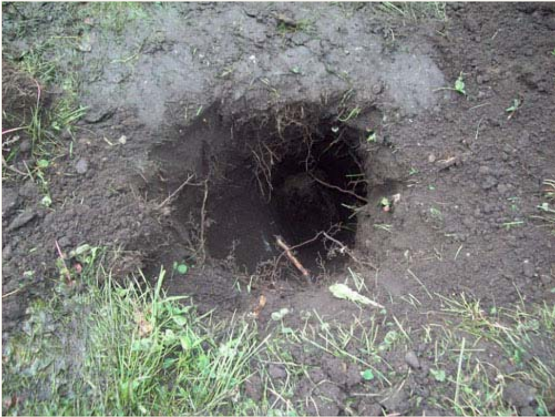
Figure 3a: Test Pit 4
