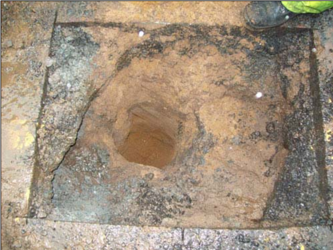
Figure 3b: Test Pit 9
