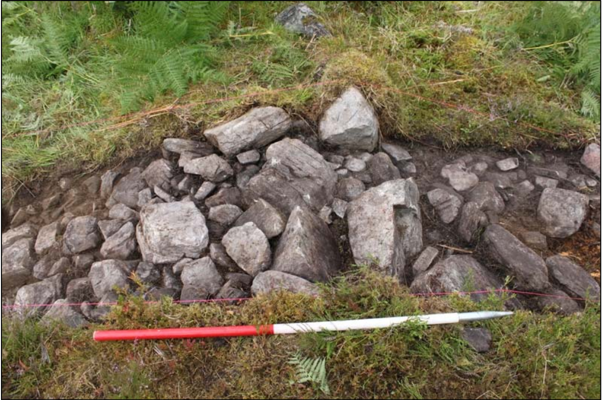
Figure 8a: Trench 3 from southeast, rubble wall prior to removal of tumble
