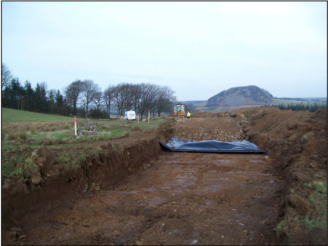
Figure 5a: Spur 1; ground reduction (construction of access road)
