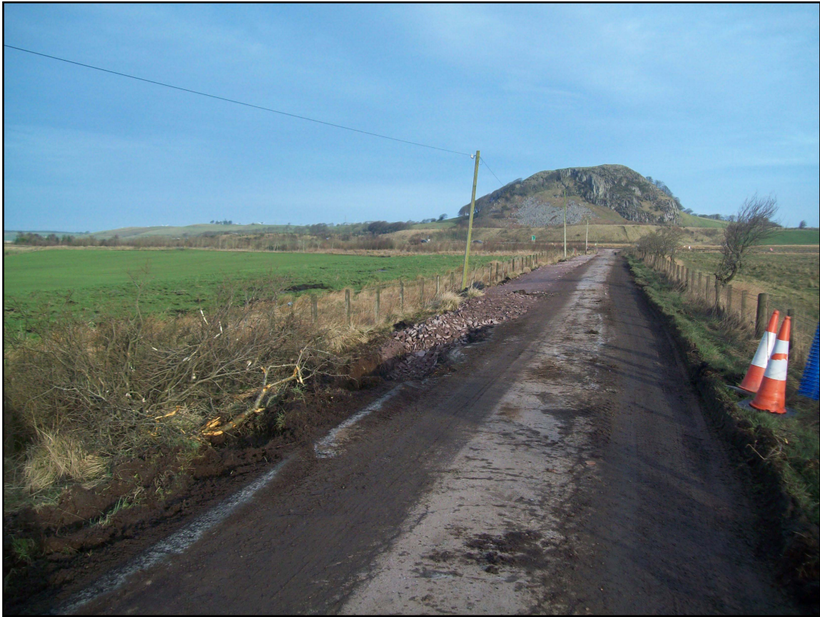
Figure 3a: Spur 1; widening of road, from CH0
