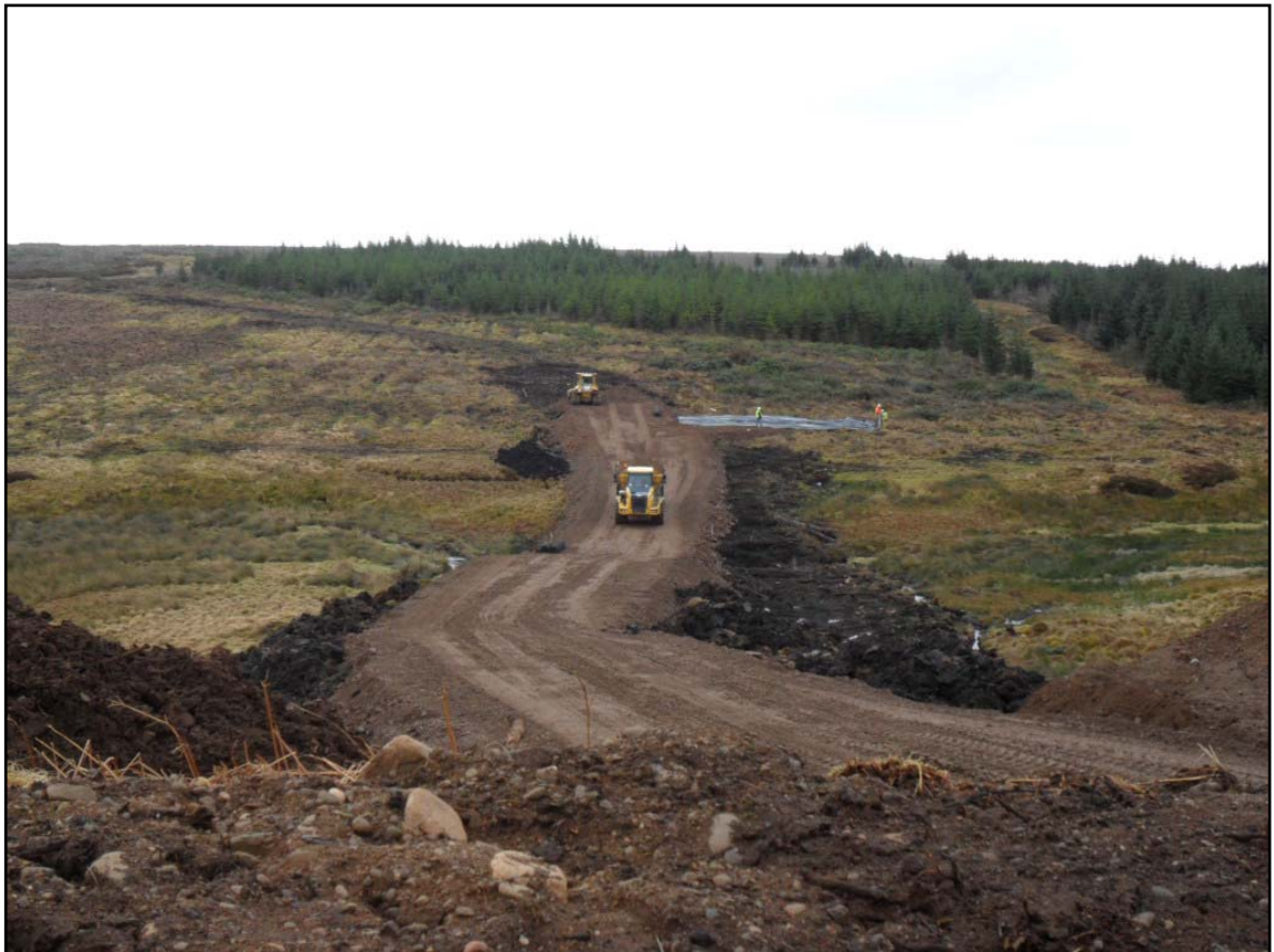
Figure 5b: Beginning of Spur 2, showing construction of access road over forestry track
