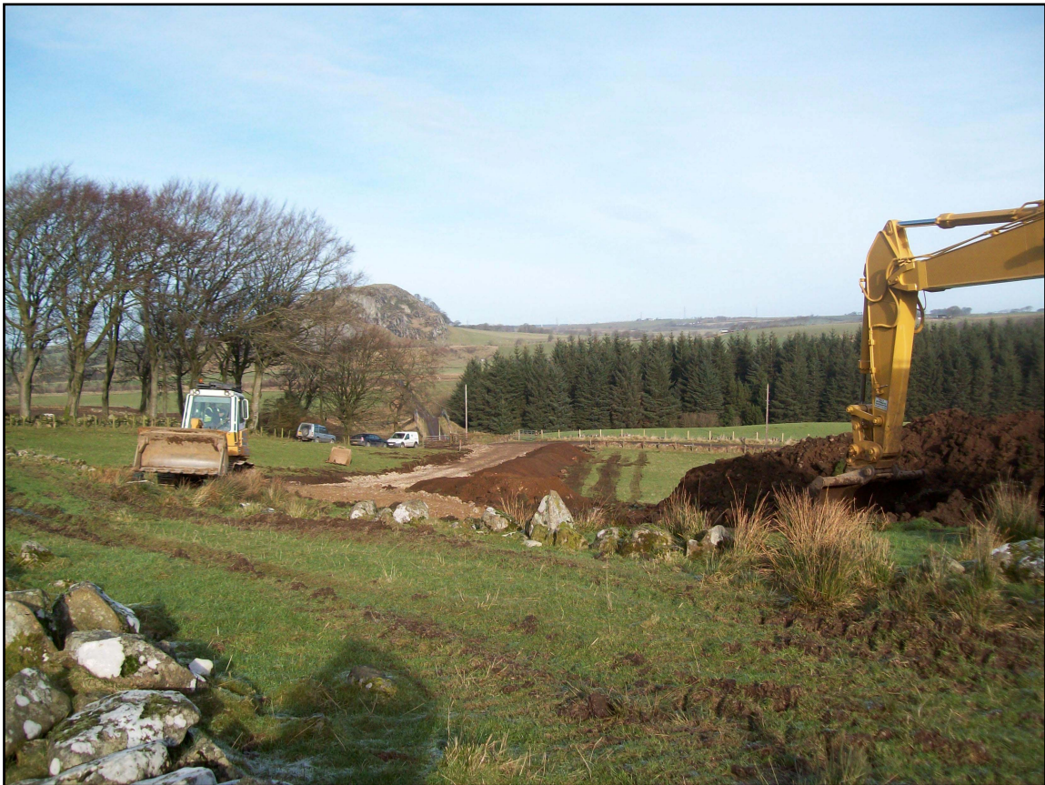
Figure 3b: Spur 1; ground reduction (construction of access road)
